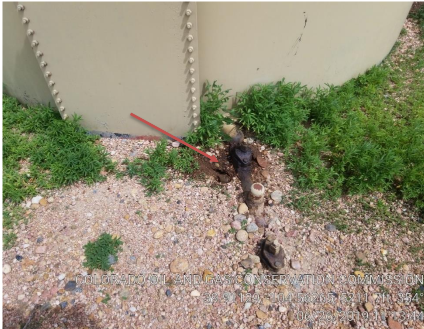
Pic 9 possible leak stained soil
