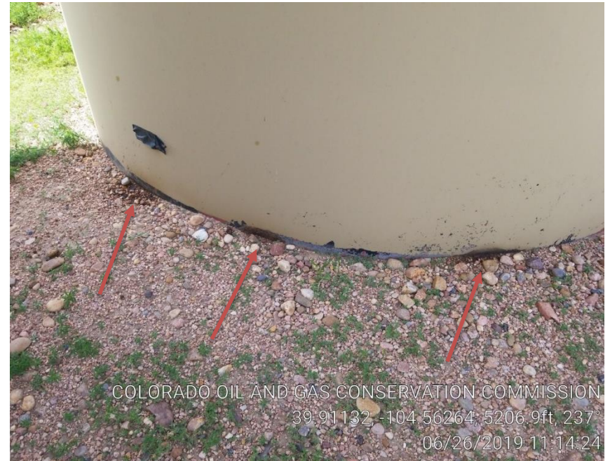
Pic 10 possible leak on bottom of tank
