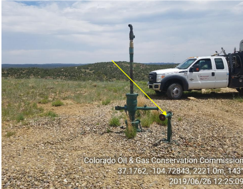
PHOTO 3: UNUSED EQUIPMENT ON LOCATION (UNUSED RISER). COMPLY WITH RULE 603.f. AND NTO REGARDING UNUSED RISERS. CA DATE 9/26/19.
