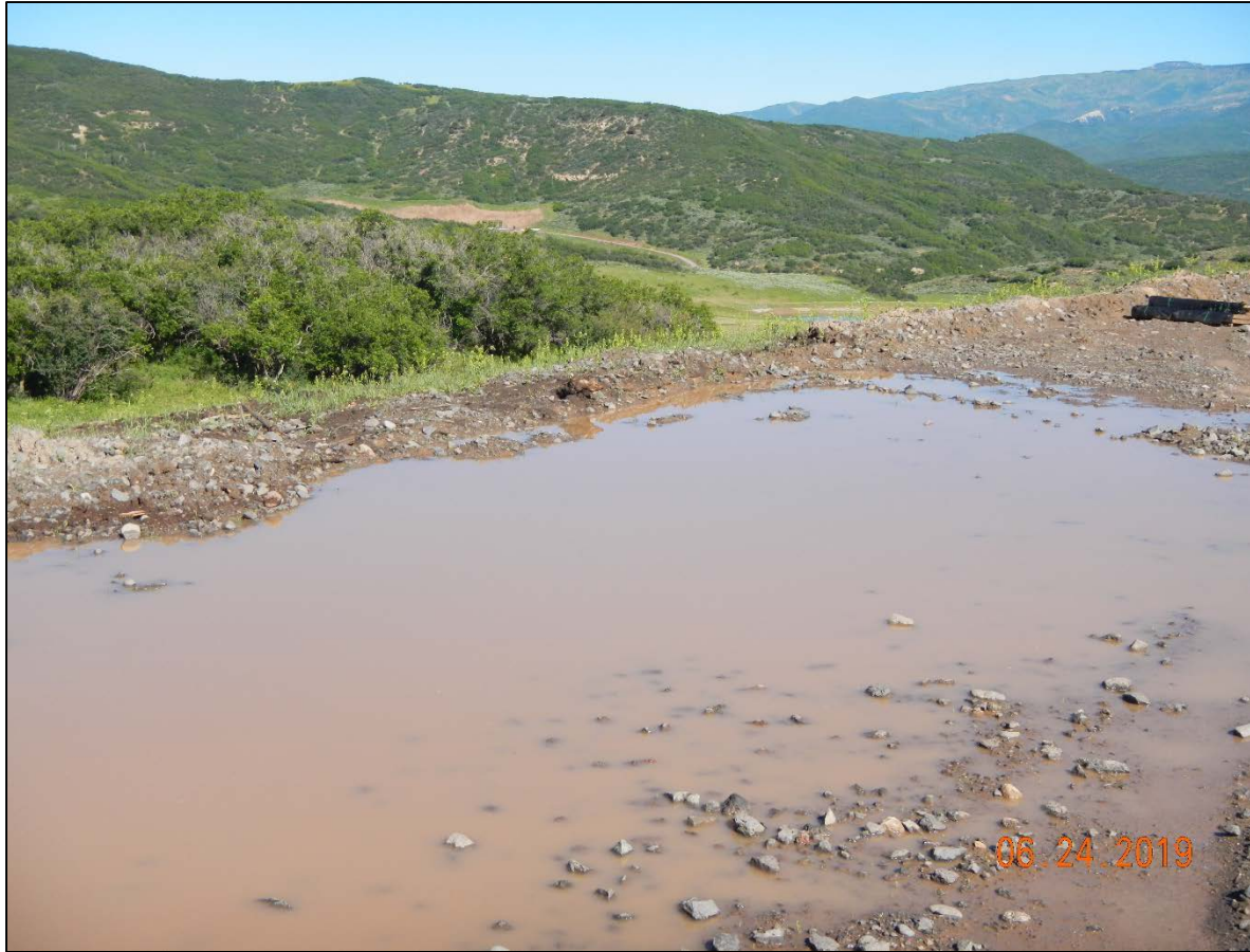
Photo #7 SW side of location BMP is damaged. Berms around location have been constructed as storm water BMP, with no stabilization, and damage.
