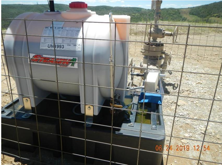
**Secondary containment of chemical container is full of fluids.**
