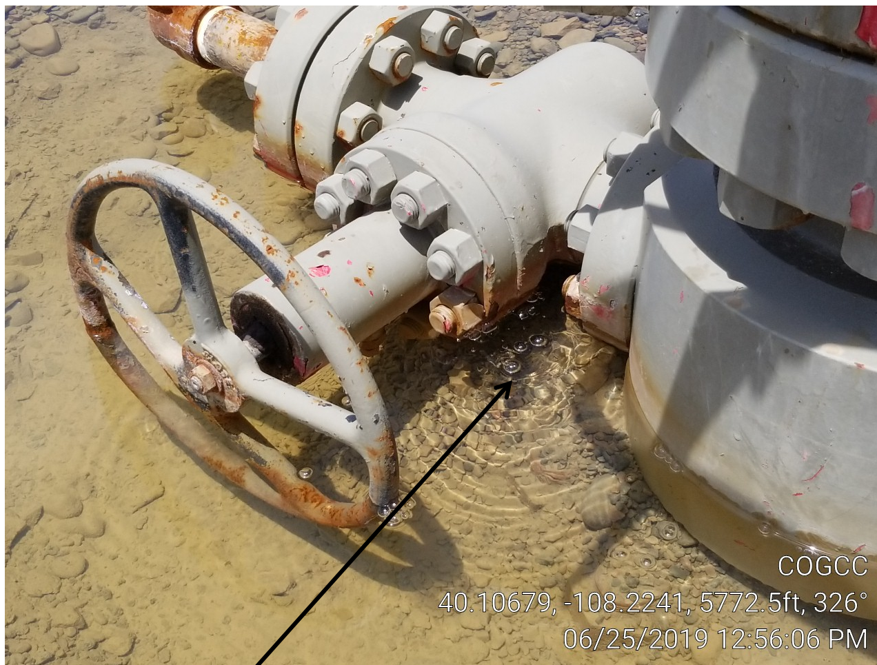
Photo 2. Gas leak on UIC well 25-43 SWD.
