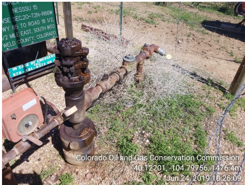
Photo 3 Mechanical issue: Packing appears to be leaking and stained soil around WH
