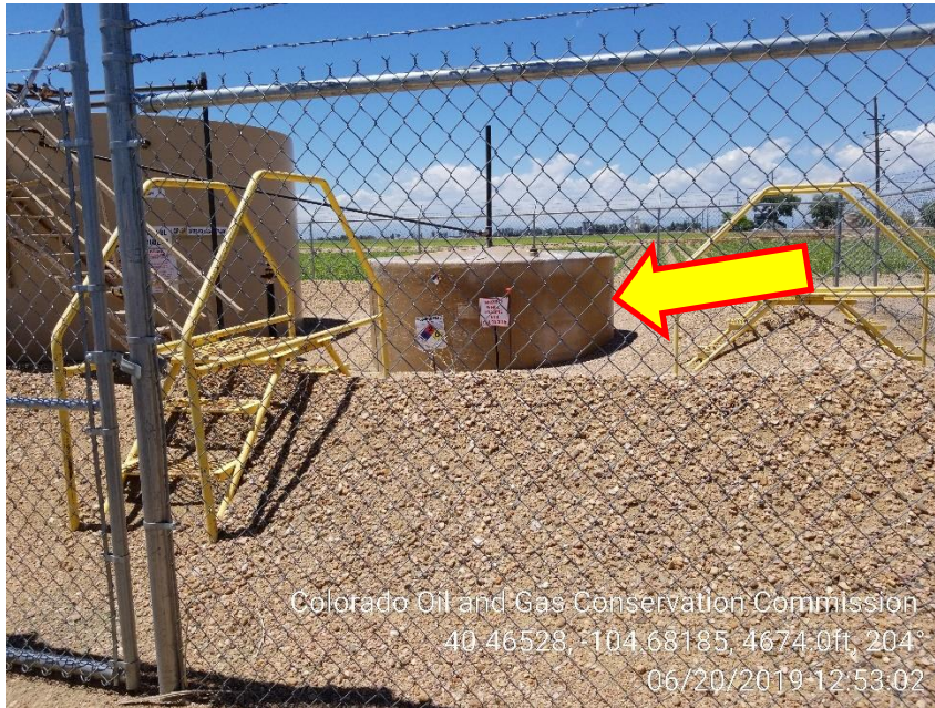
Photo 3 – Produced Water Vault missing Capacity Contents
