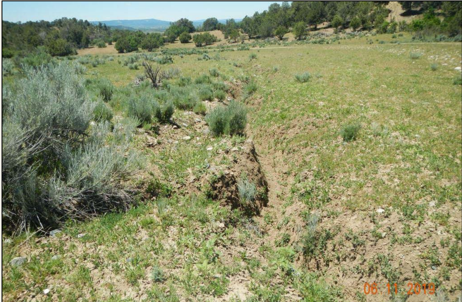
Photo 3. View of head-cut erosion and erosional channeling downstream from culvert outlet along the access road. This appears to be a result of concentrated stormwater flows exiting the culvert.
