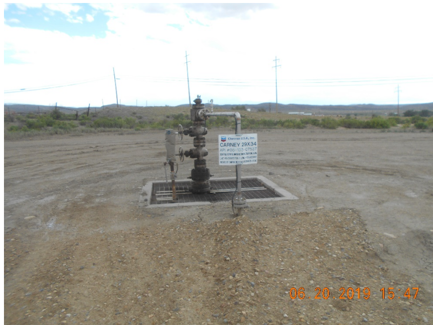
Injection wellhead
