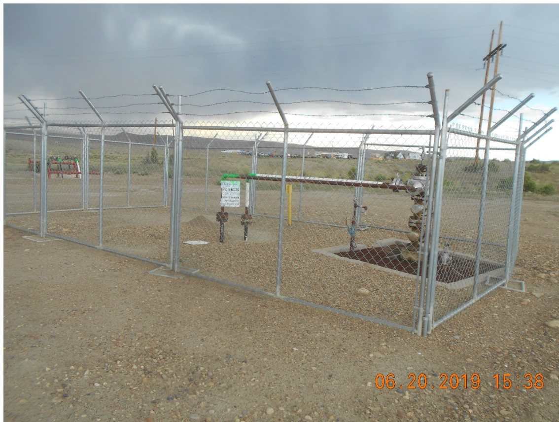
Injection wellhead
