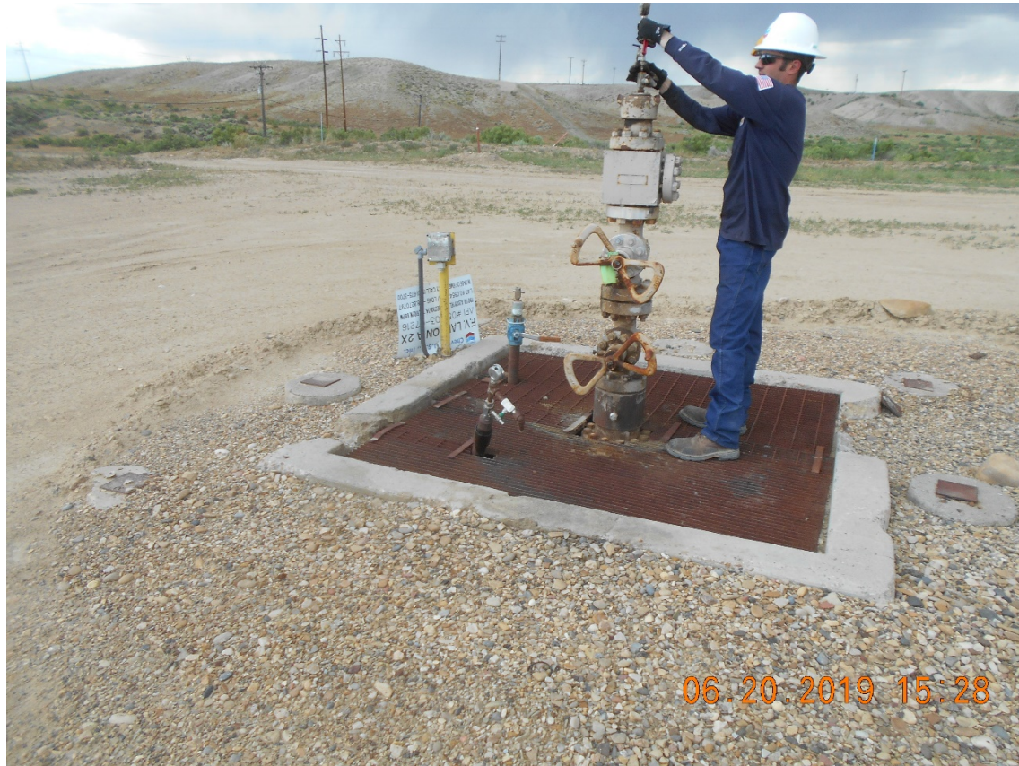
Injection wellhead
