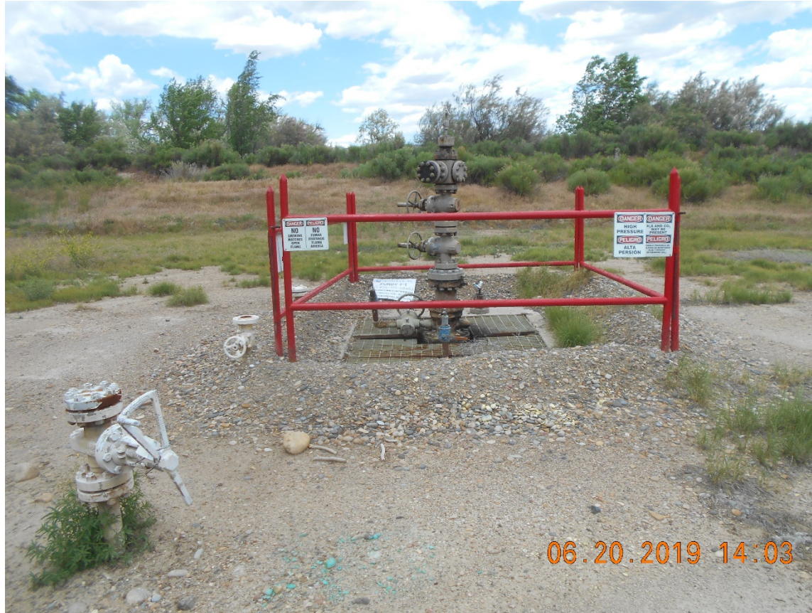
Injection wellhead – Temporarily abandoned
