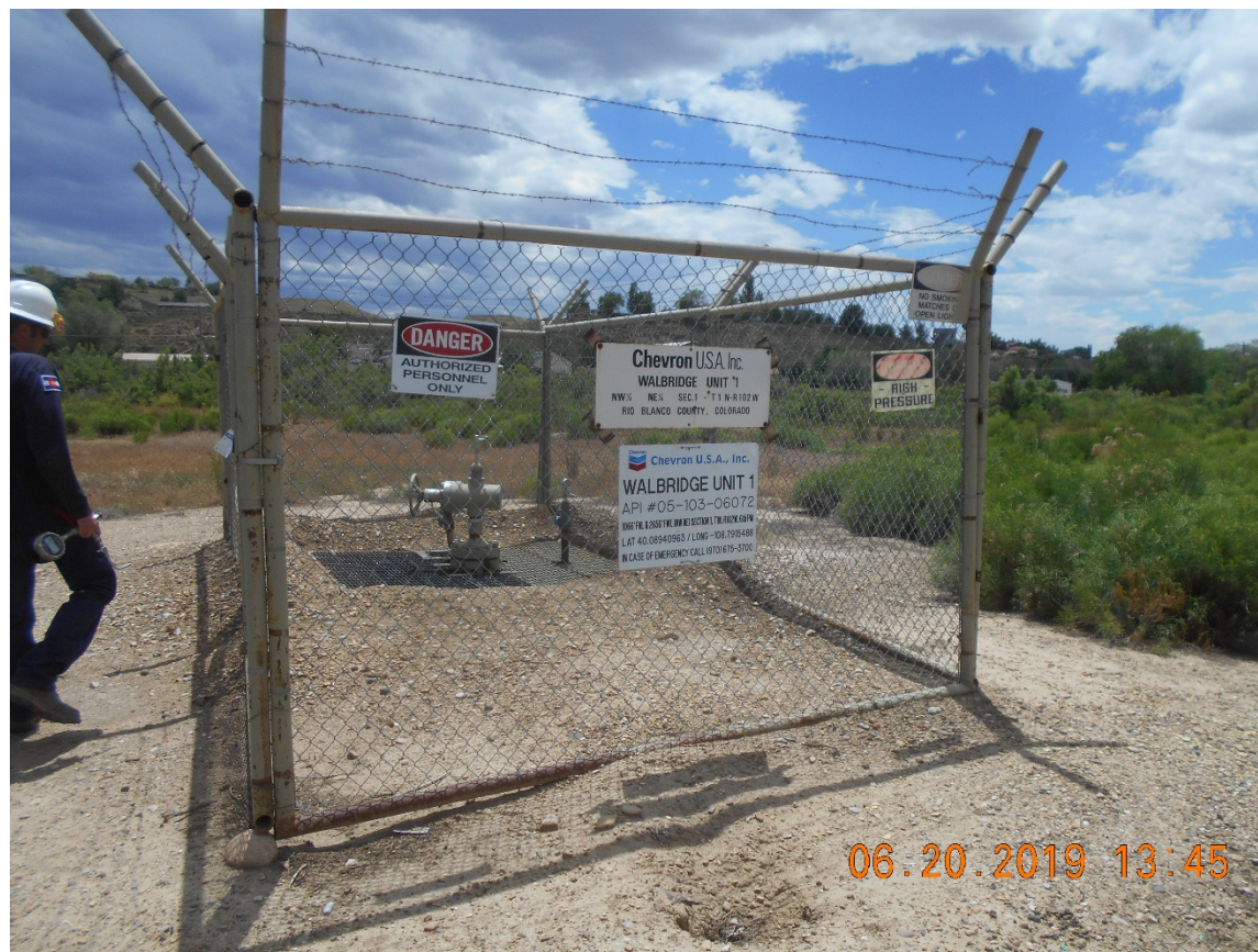
Injection wellhead – Temporarily abandoned
