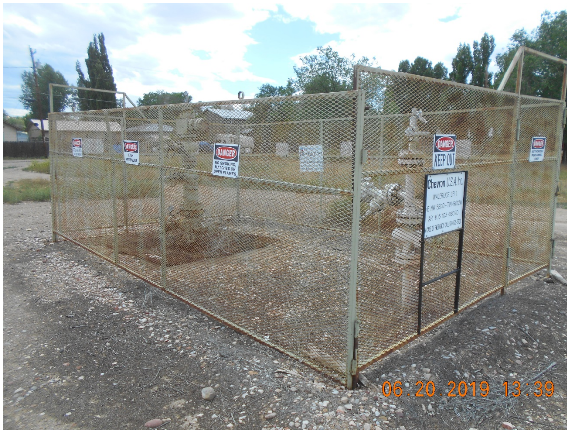
Injection wellhead – Temporarily abandoned
