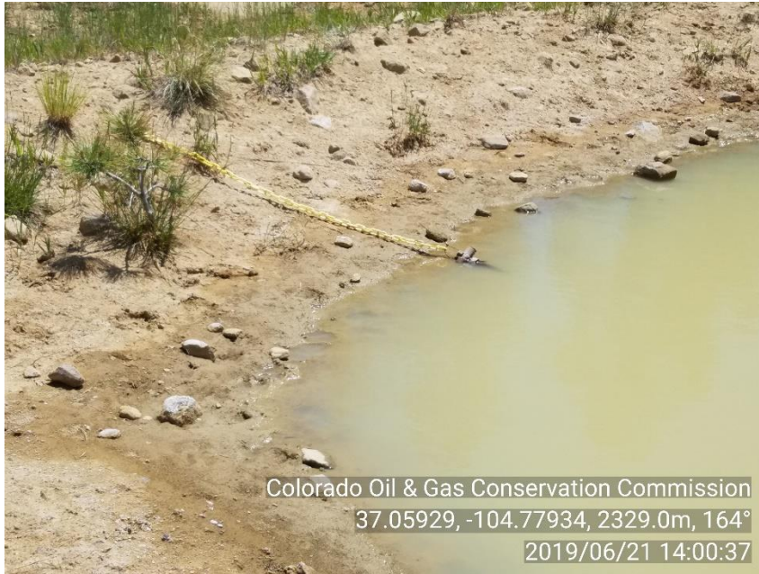
PHOTO 3: PRODUCED WATER LEVEL IN PIT IS AT FREEBOARD MARKER. CALL ANSWERING SERVICE AND LEFT MESSAGE TO HAVE ON CALL PERSONEL CALL ME BACK. LOWER FLUID LEVEL IN PIT SO THAT AT LEAST 2' FREEBOARD IS MAINTAINED AT ALL TIMES PER RULE 902.b. CA DATE 6/22/19
