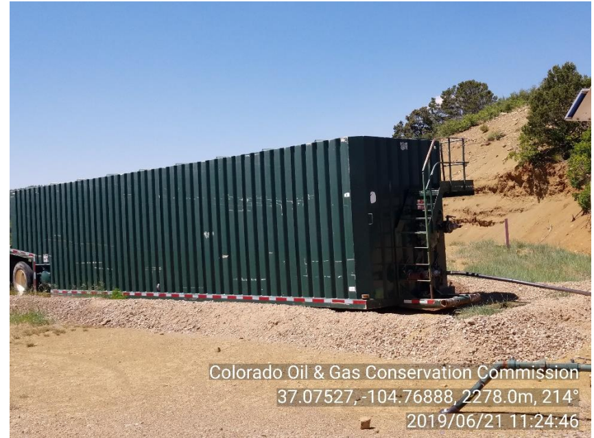
PHOTO 6: NO NFPA STICKER POSTED ON PRODUCED WATER TANK. ALSO CAPACITY OF TANK IS NOT POSTED. COMPLY WITH RULE 210. d.
