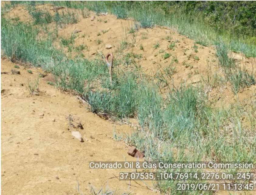
PHOTO 7: GUY LINE ANCHOR NOT MARKED. INSTALL GUY LINE MARKER IN ACCORDANCE WITH RULE 1003.a.
