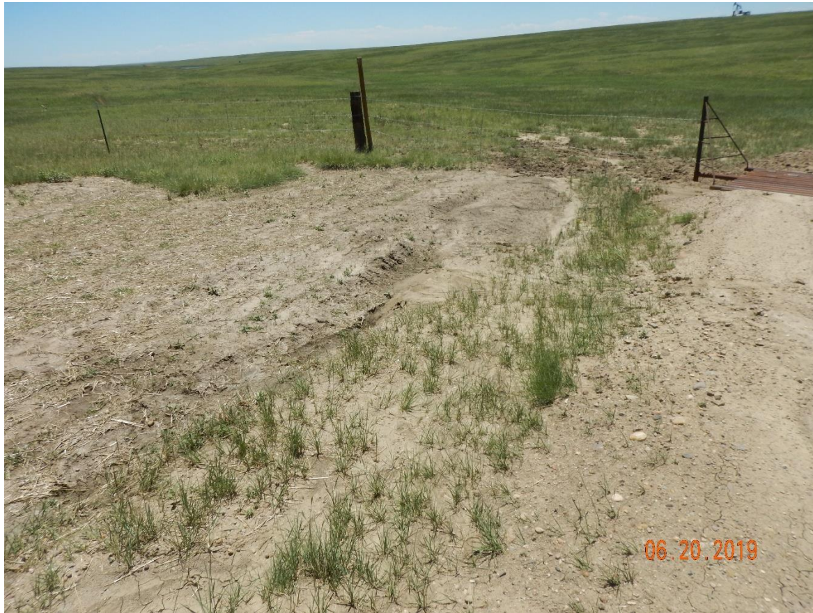
Photo 4: Photo taken from the southwest end of the location, facing southwest. Photo shows stormwater runoff is beginning to cause erosion degradation with sediment discharge onto the adjacent lands. Advise installing BMPs
