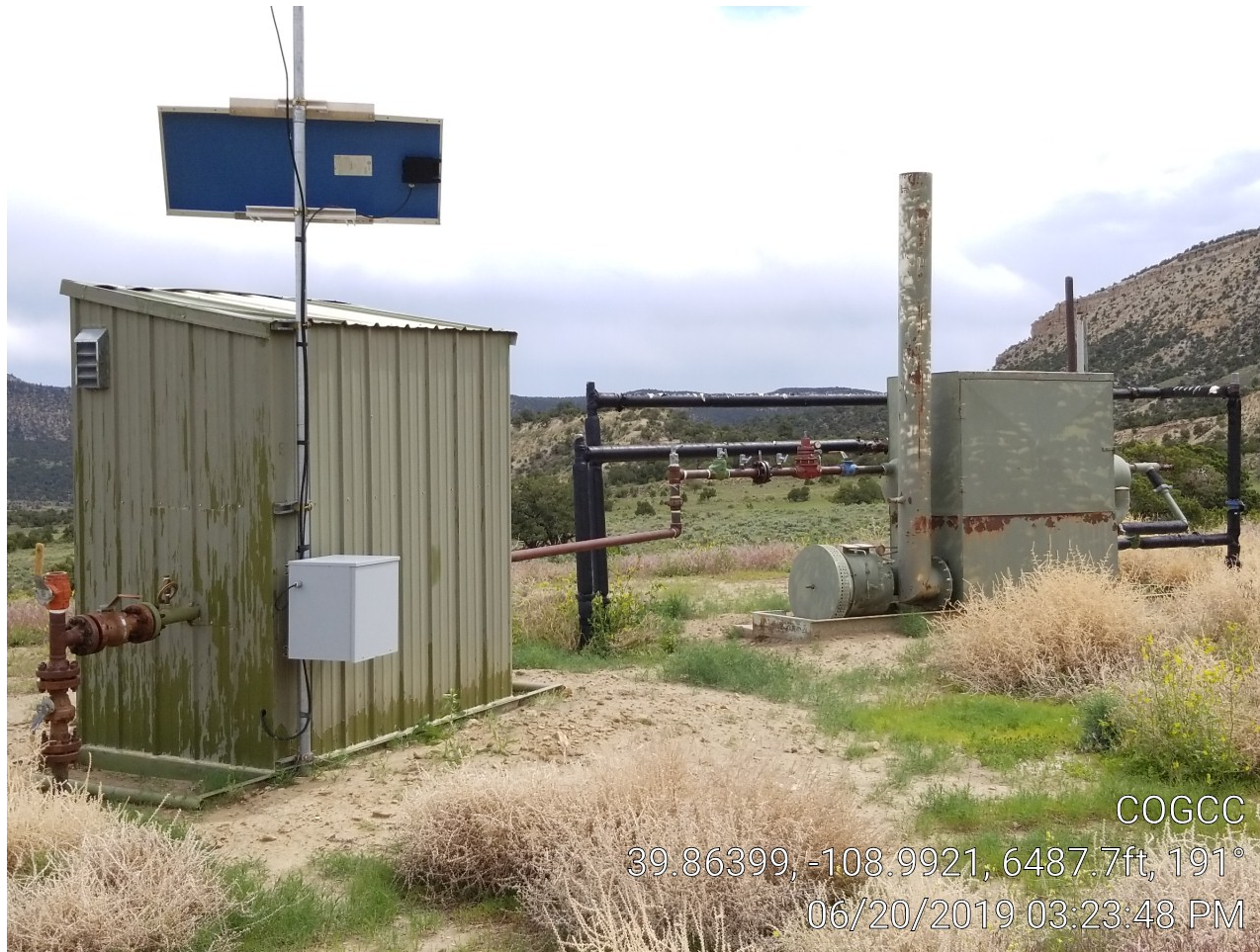
Photo 3. Meter building & separator.
