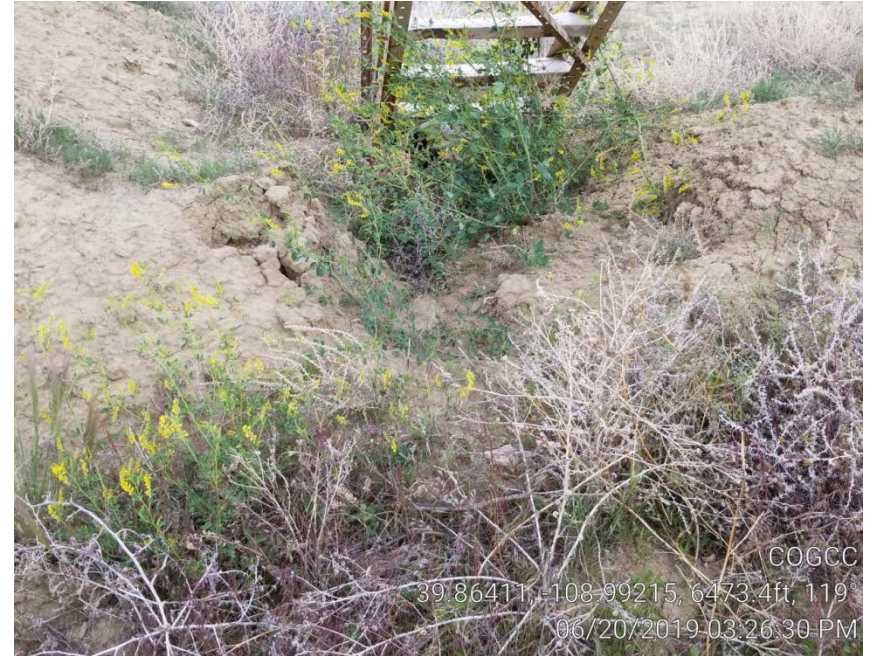
Photo 8. Erosion channel exiting tank battery secondary containment. Also weeds on berm.
