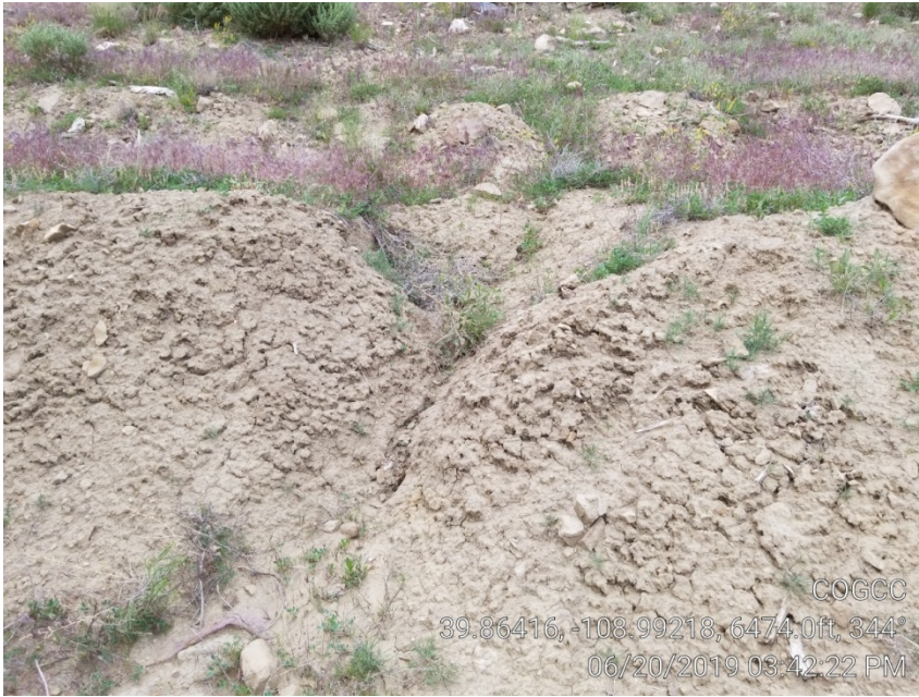
Photo 7. Erosion channel entering tank battery secondary containment.
