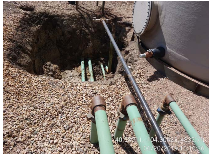
Photo 2 – Photo of dumplines and adjacent excavation at rear of produced water fiberglass AST.
