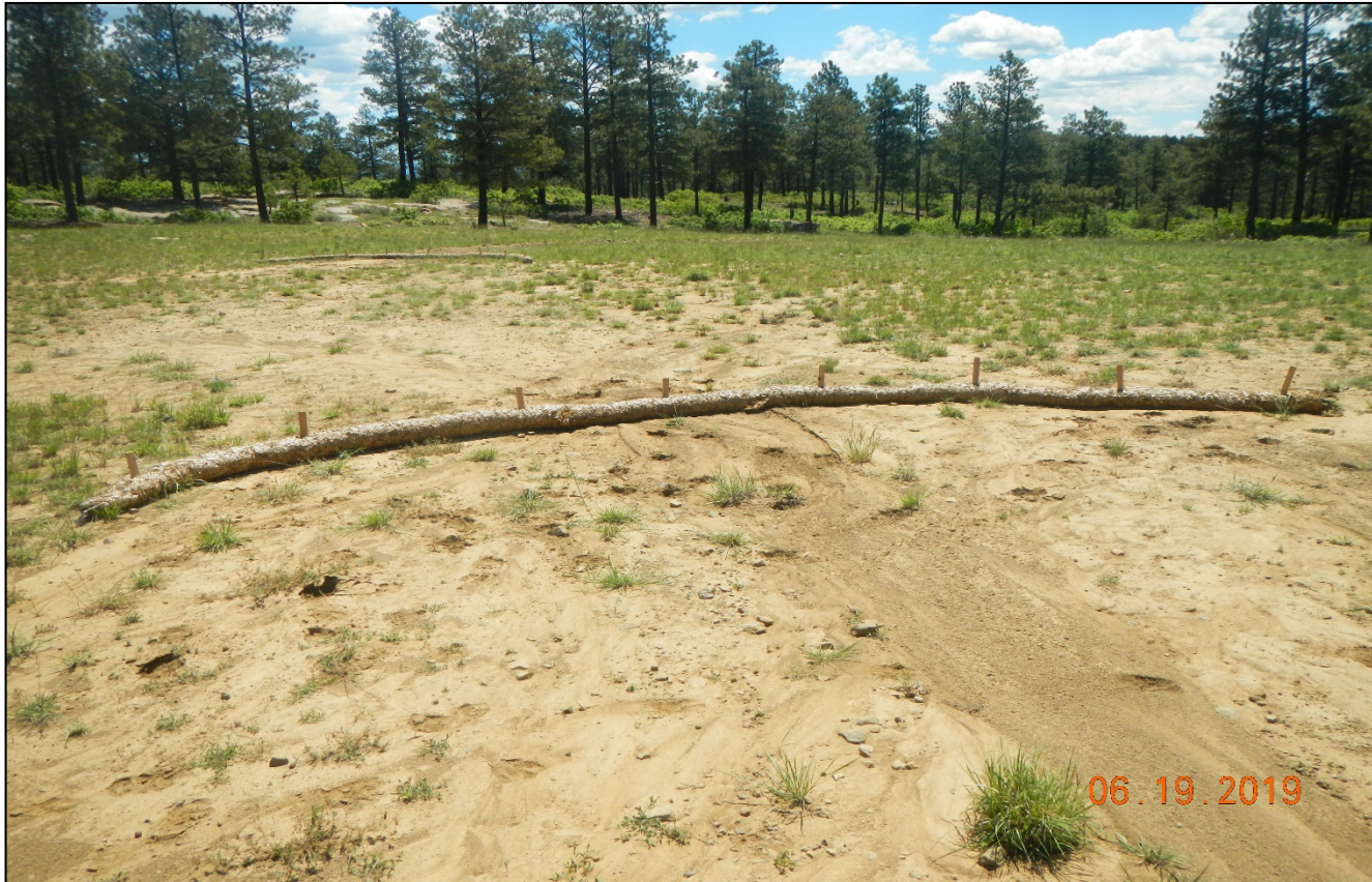
Photo 3. Wattles were installed. There was no sign of seeding or germination in area. Erosion may have washed away seed.
