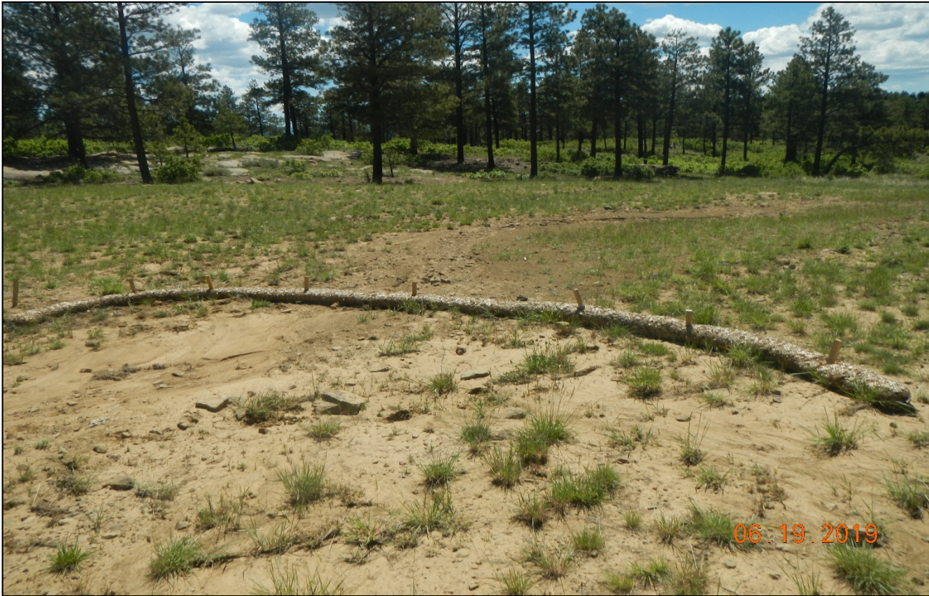
Photo 4. Wattles have been installed however stormwater is flowing underneath wattles.,
