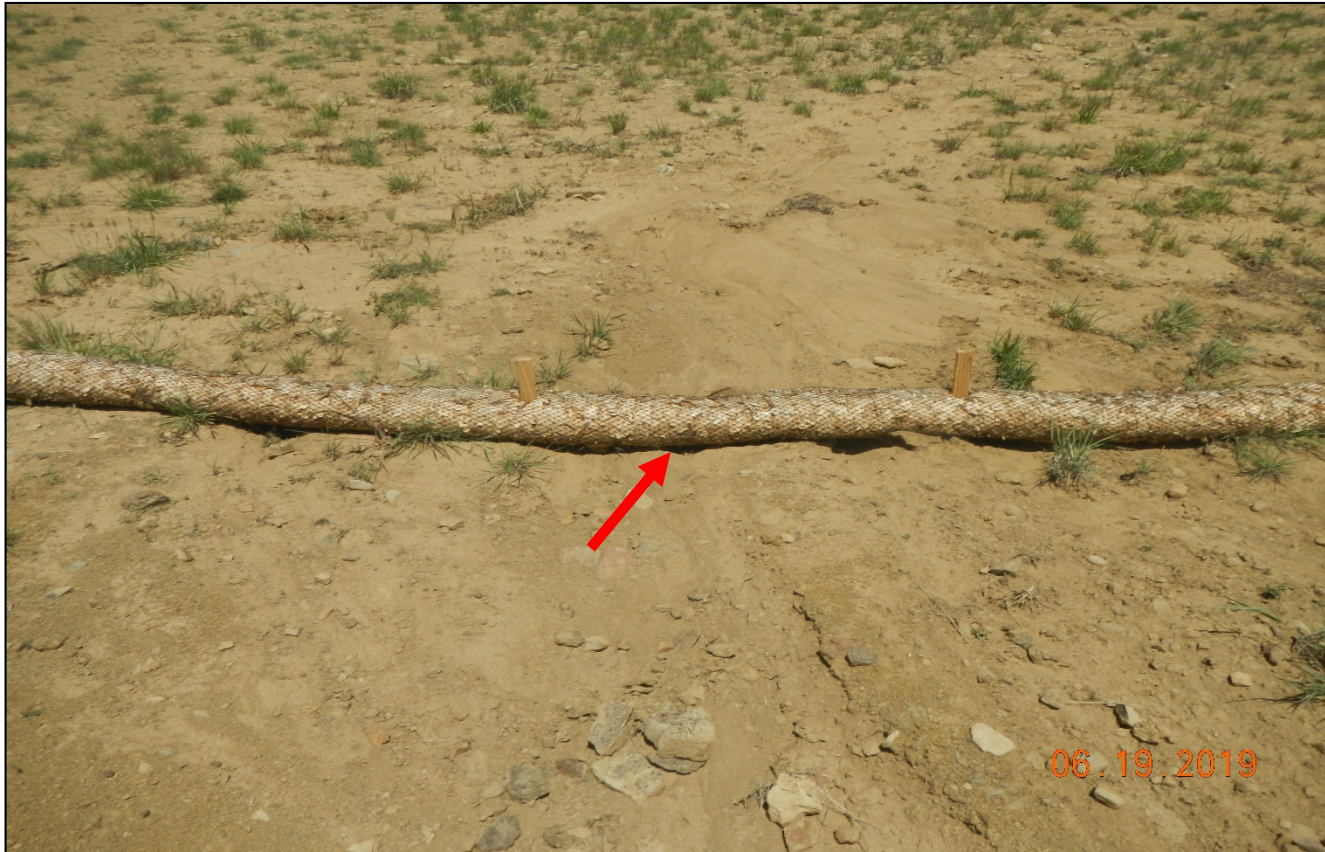
Photo 5. There are sign stormwater is flowing underneath the wattle. Wattles were not properly trenched into the ground.
