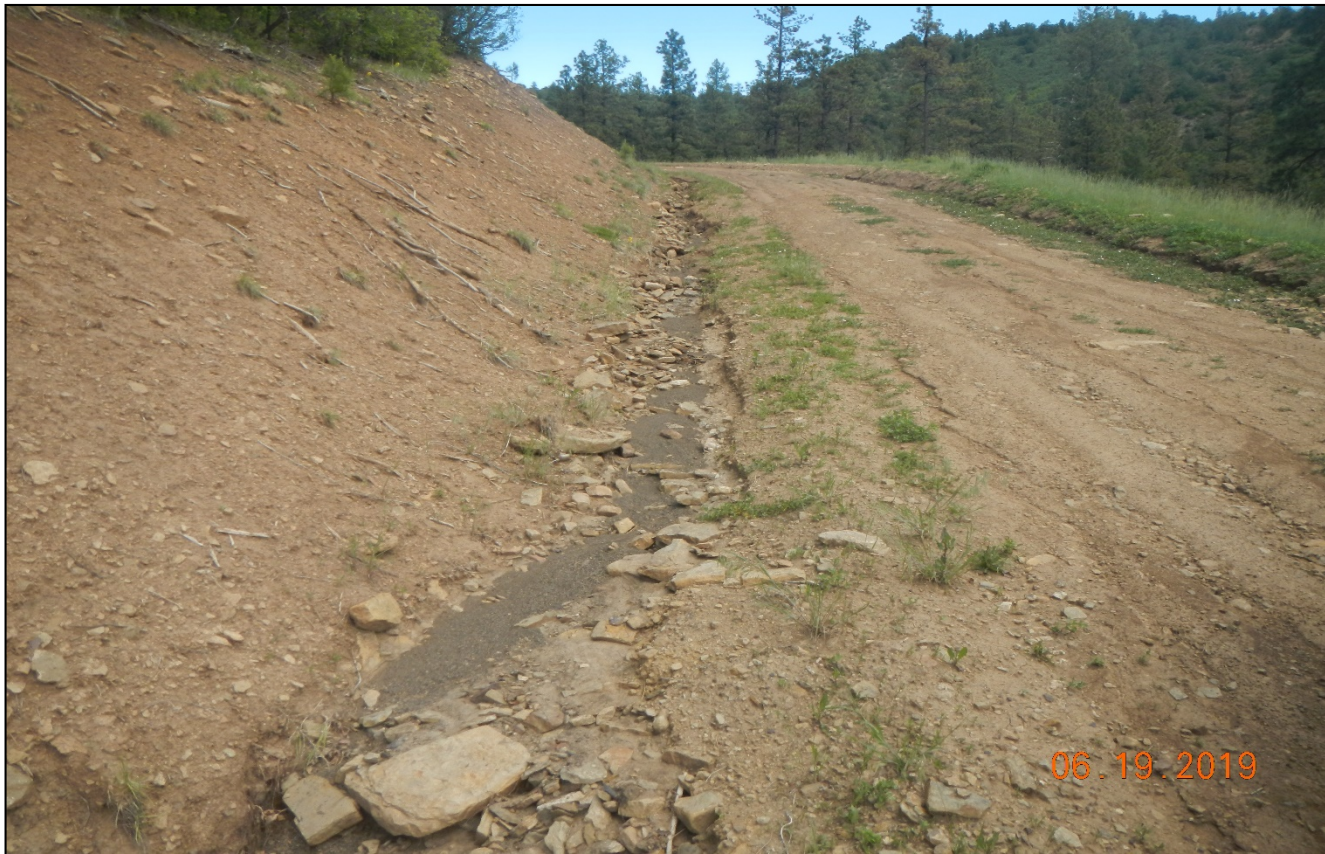
Photo 2. There is erosion down the side of the road. No BMPs installed to prevent erosion. Lat/Long:37.02576,-104.83253
