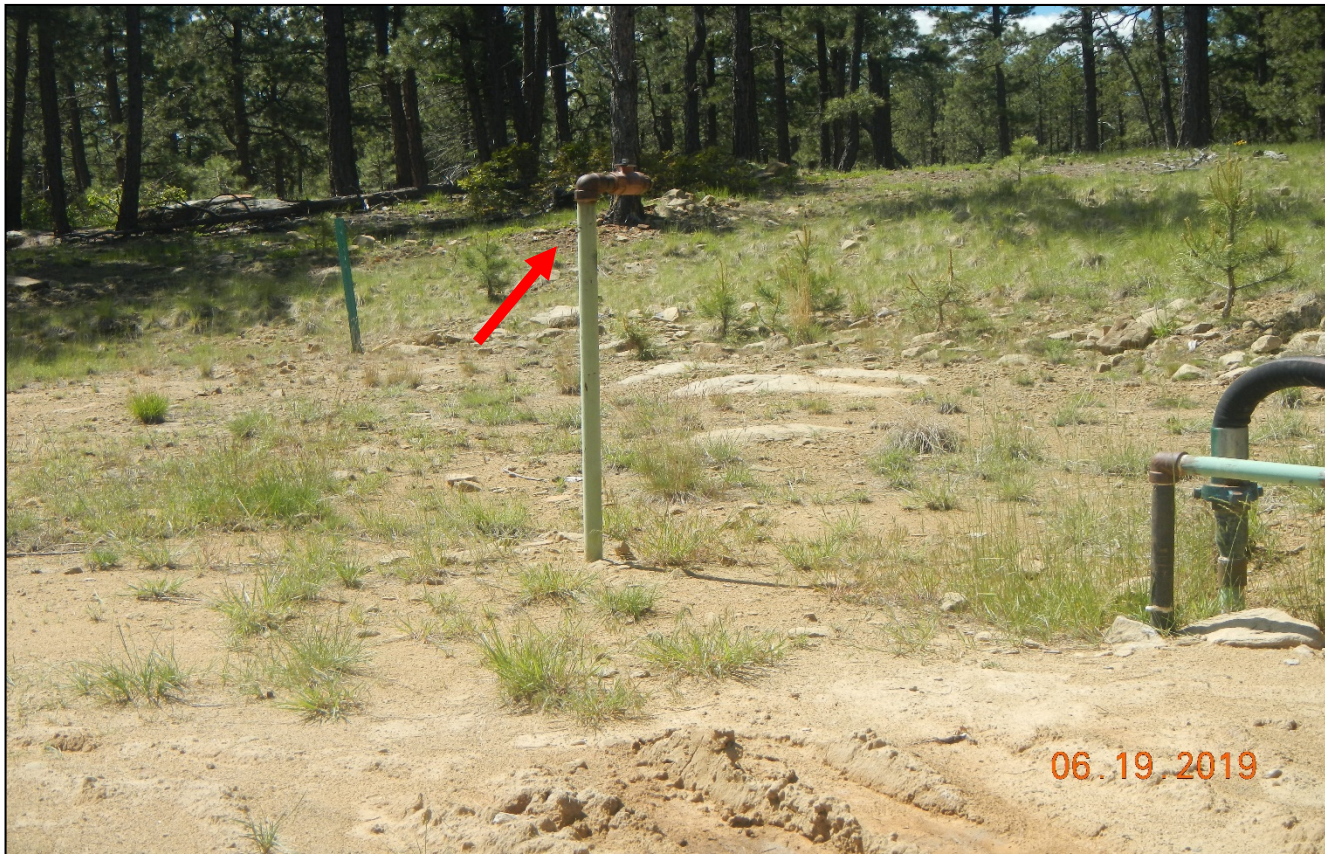
Photo 5. No LO/TO on pipe riser.
