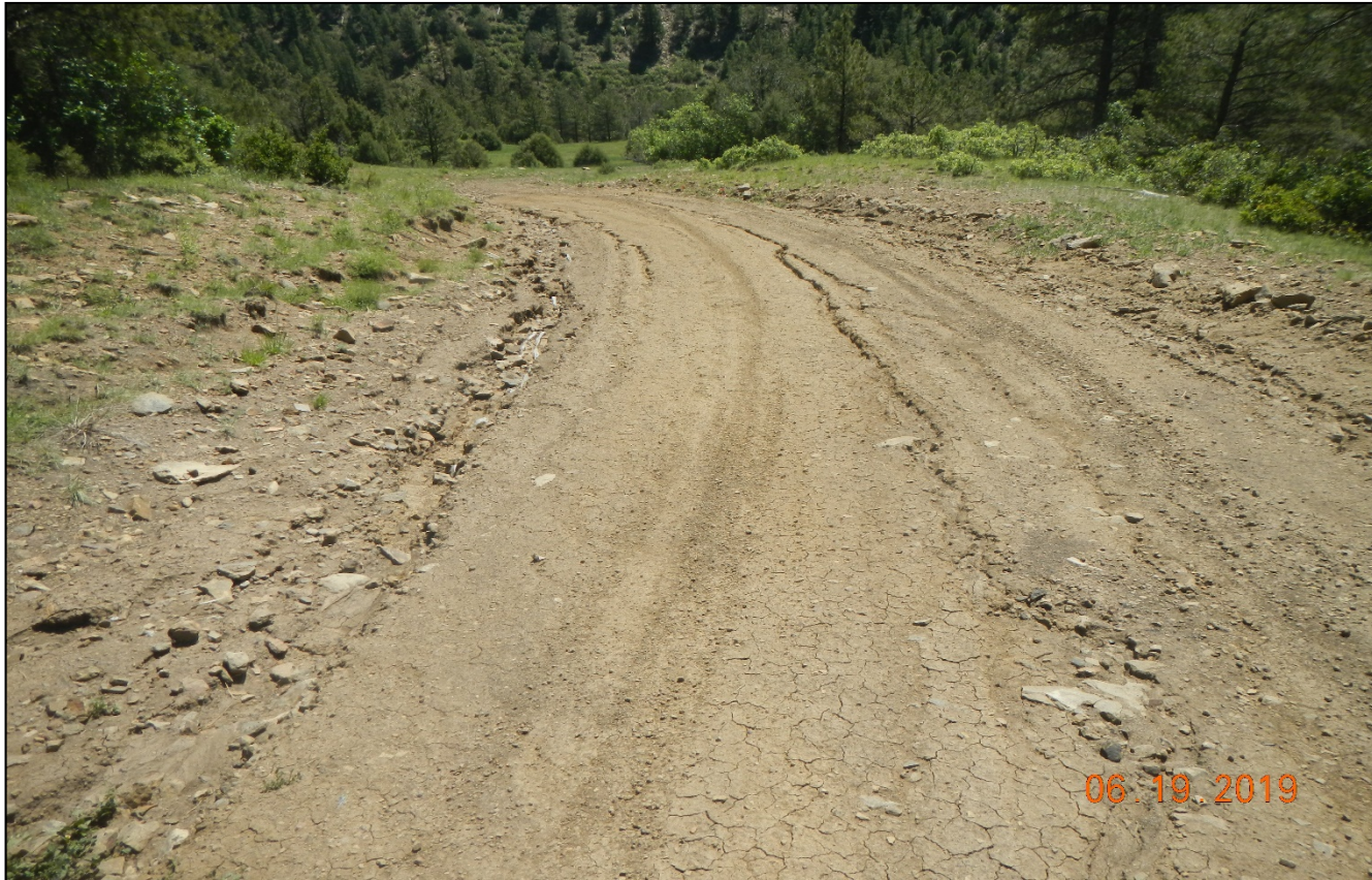
Photo 2. There is erosion occurring down the road and no BMP's are installed.
