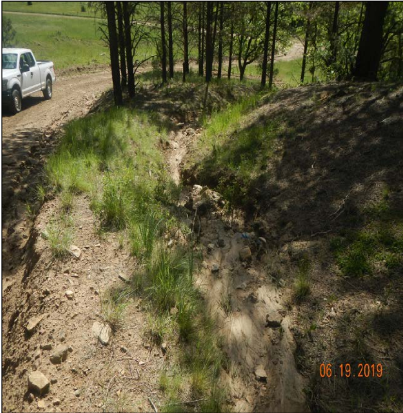
Photo 2. These two diversion ditches are transporting sediment offsite. No BMP's installed. Sediment trap or check dams would prevent sediment transport offsite.
