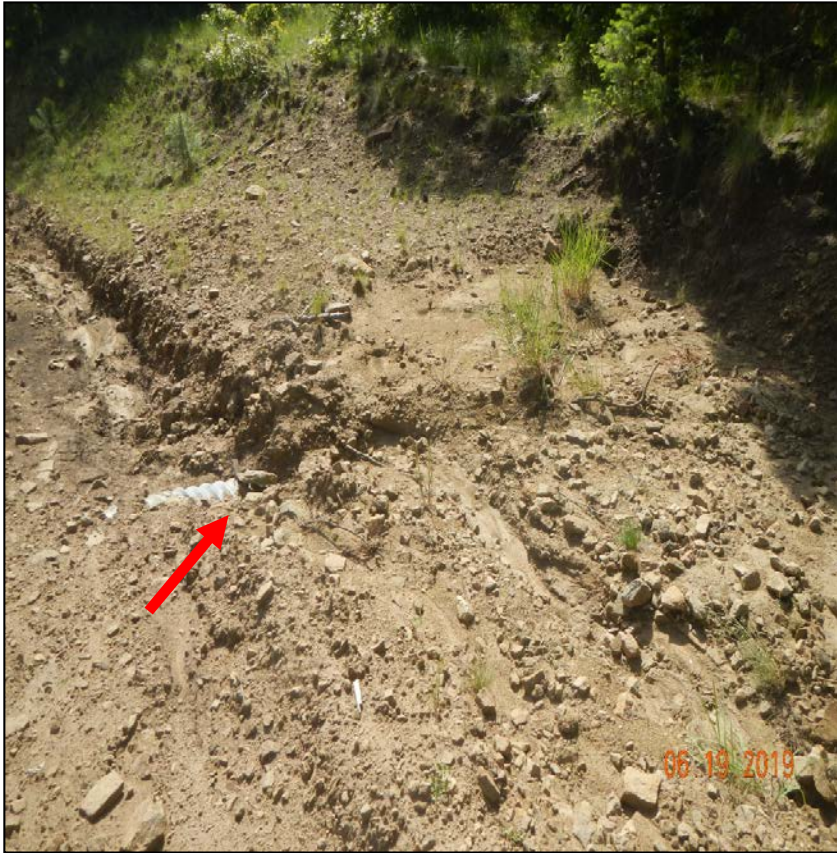
Photo 4. The photo on left is culvert inlet filled with sediment. Photo right is damaged culvert near outlet. Lat/Long:37.00845,-104.84245
