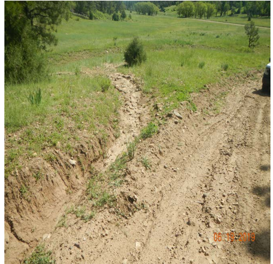
Photo 2. These two diversion ditches are transporting sediment offsite. No BMP's installed. Sediment trap or check dams would prevent sediment transport offsite.
