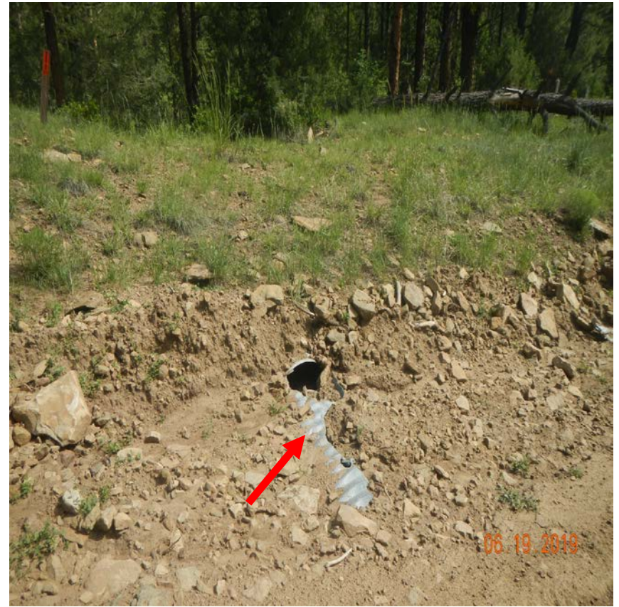
Photo 4. The photo on left is culvert inlet filled with sediment. Photo right is damaged culvert near outlet. Lat/Long:37.00845,-104.84245
