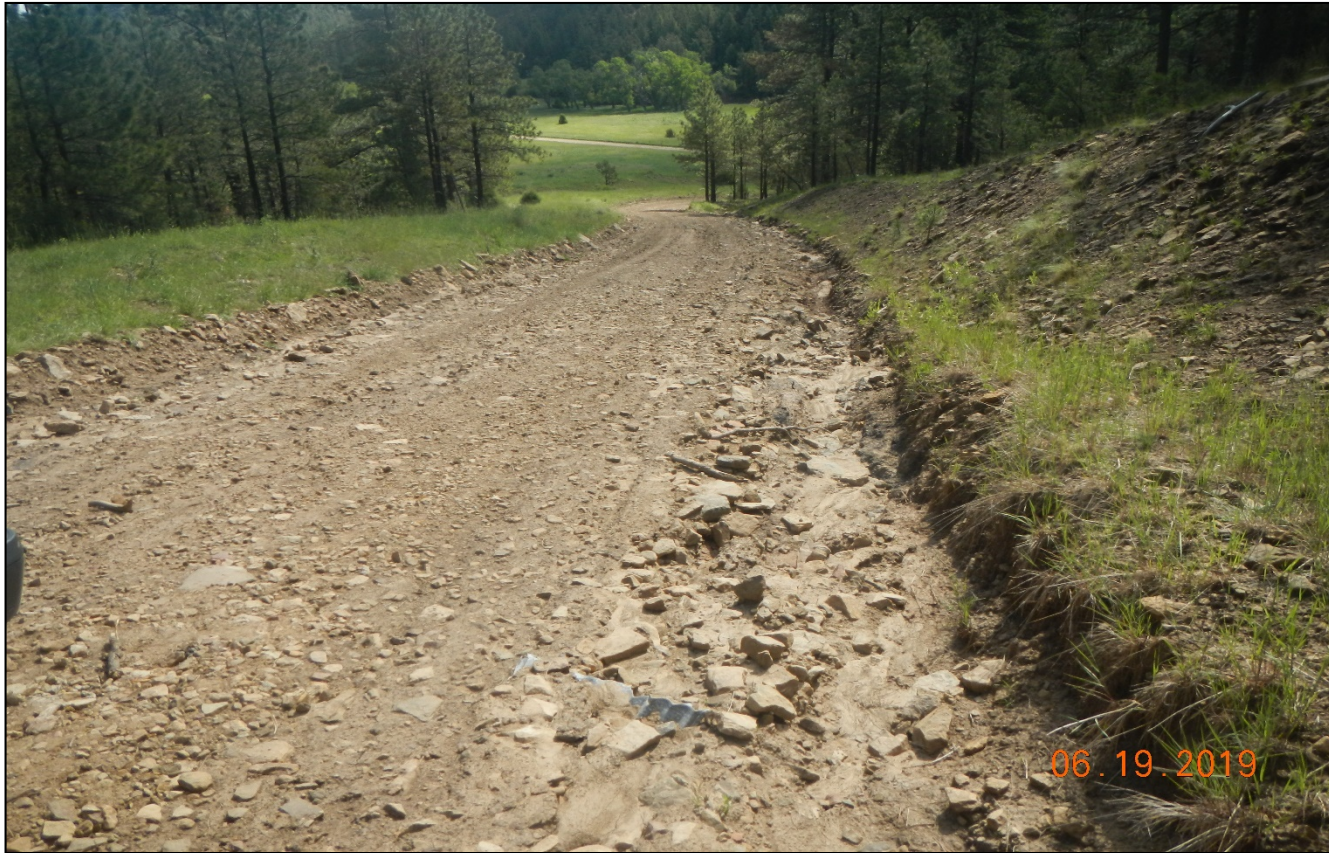
Photo 3. Stormwater is running down the road and is scouring the road. No BMP's installed.
