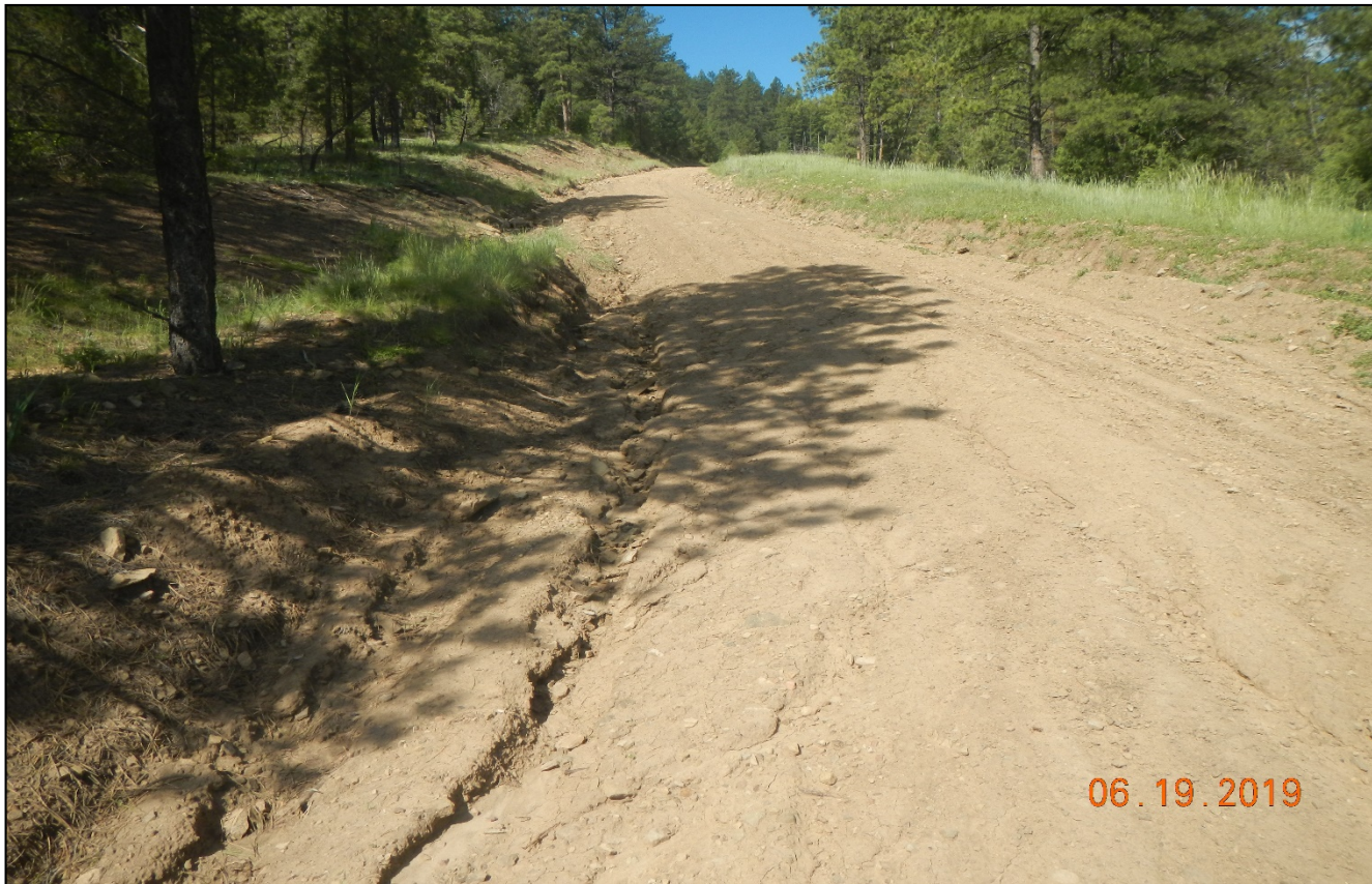
Photo 1. Stormwater is flowing down the road causing erosion.
