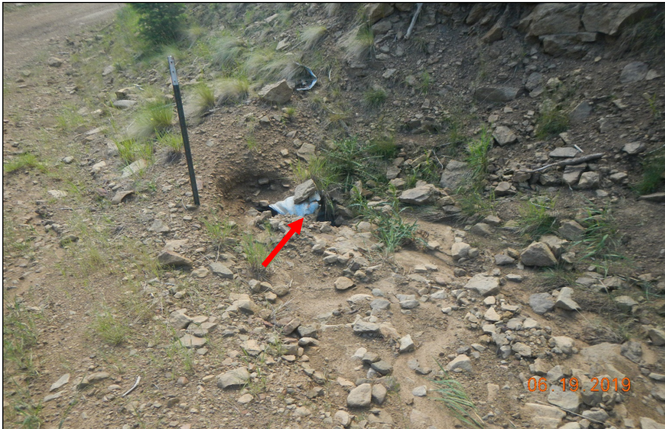
Photo 5. This culvert is filled in with sediment and damaged.
