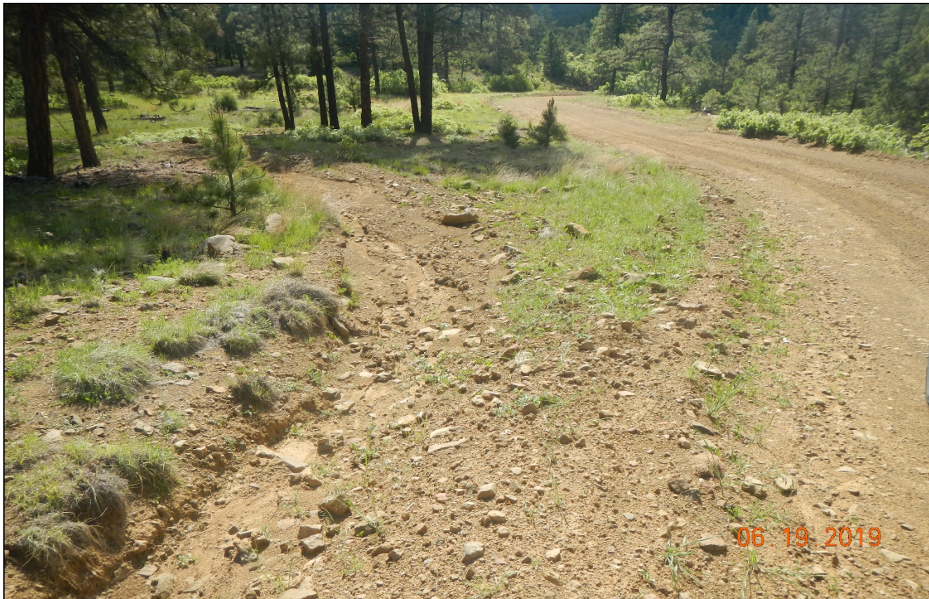
Photo 6. This diversion ditch is transporting sediment off site. No BMP's installed.
