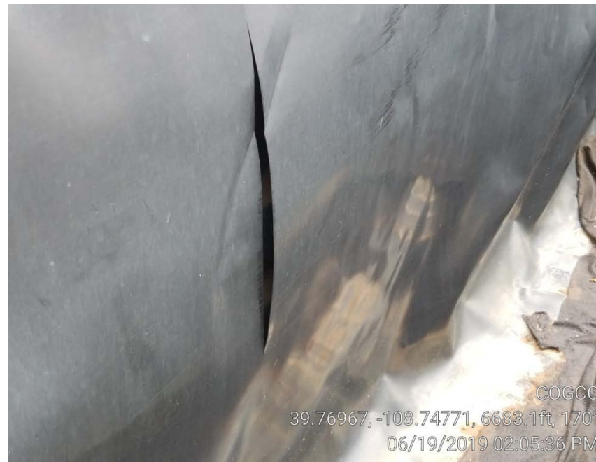
Photo 3. Tank liner tear.
