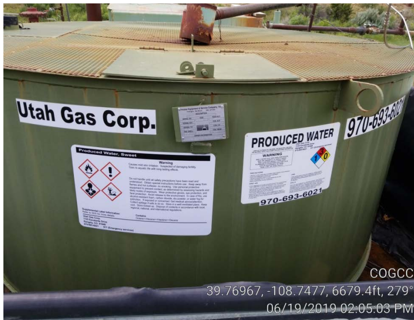
Photo 2. Missing tank capacity label.
