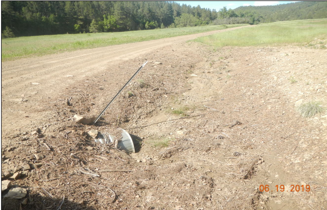
Photo 1. The culvert along the main road has filled in with sediment. Lat/Long:37.02493,-104.82831
