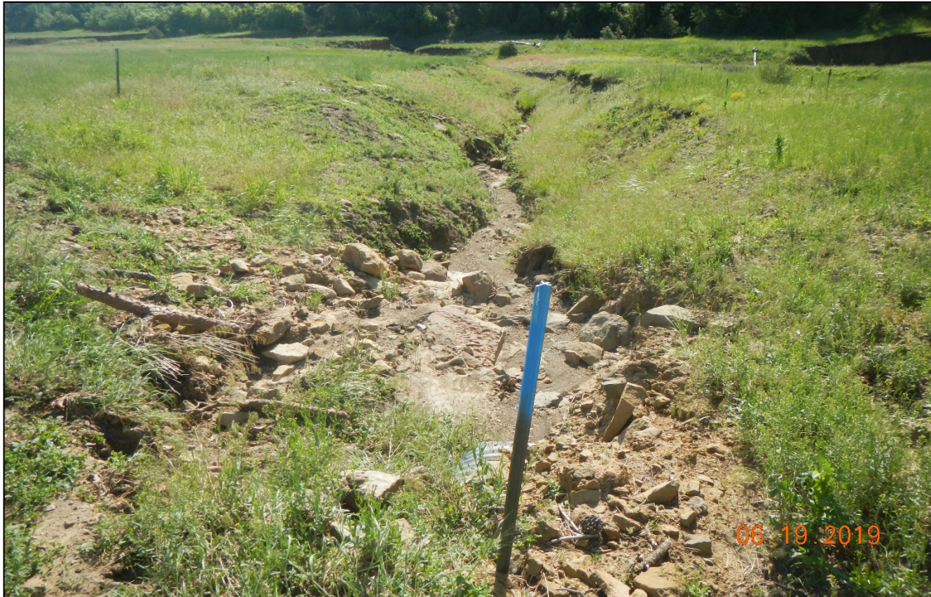
Photo 2. There is erosion occurring at the outlet culvert. No BMPs installed for outlet protection or to prevent erosion. Lat/Long:37.02425,-104.82919
