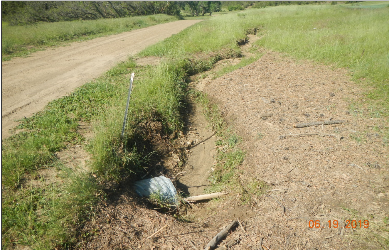
Photo 3. The culvert along the main road has filled in with sediment. Lat/Long:37.02425,-104.82919
