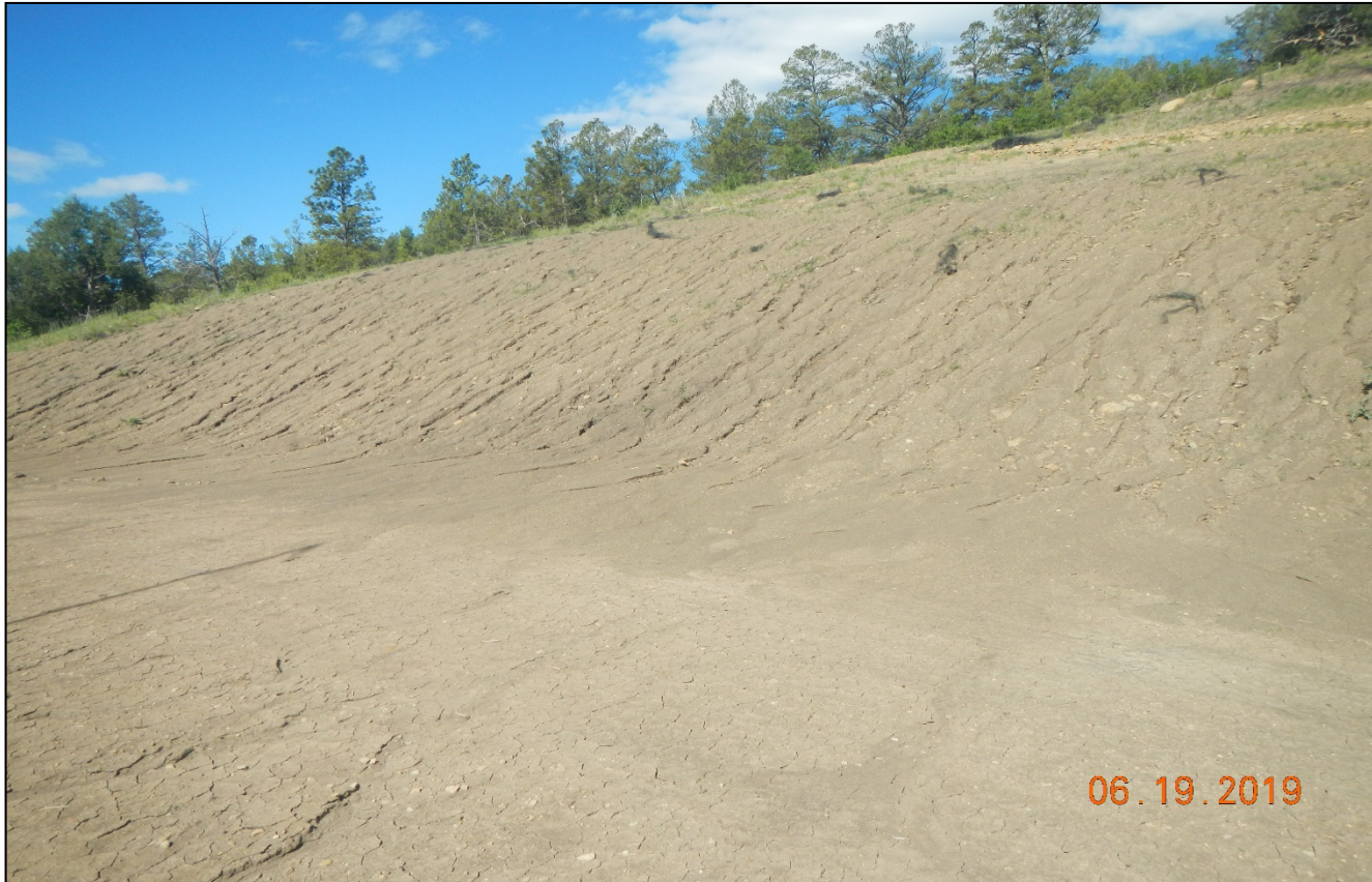
Photo 6. The cut slope is not stabilized and erosion is occurring. No vegetation is establishing.
