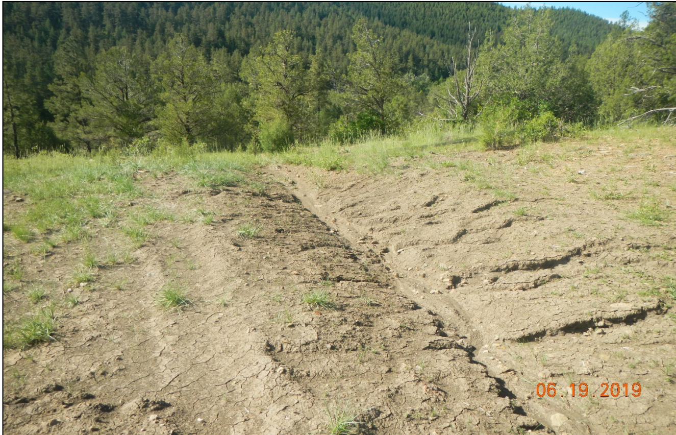
Photo 7. A diversion ditch at the southwest side is directing sediment off location. Sediment trap or other BMP is needed to prevent sediment erosion from leaving site.
