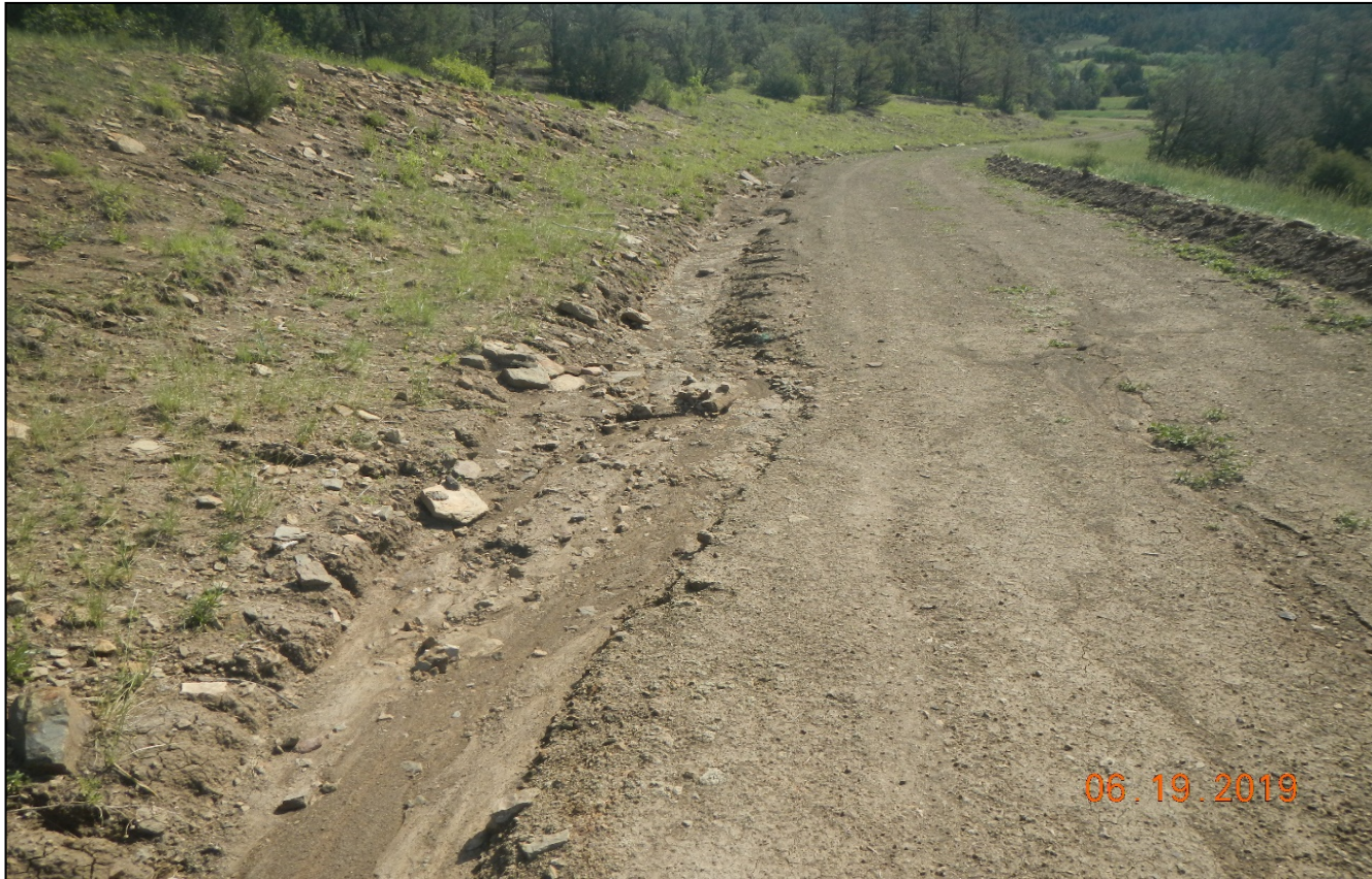
Photo 3. Stormwater erosion is occurring down the access road.
