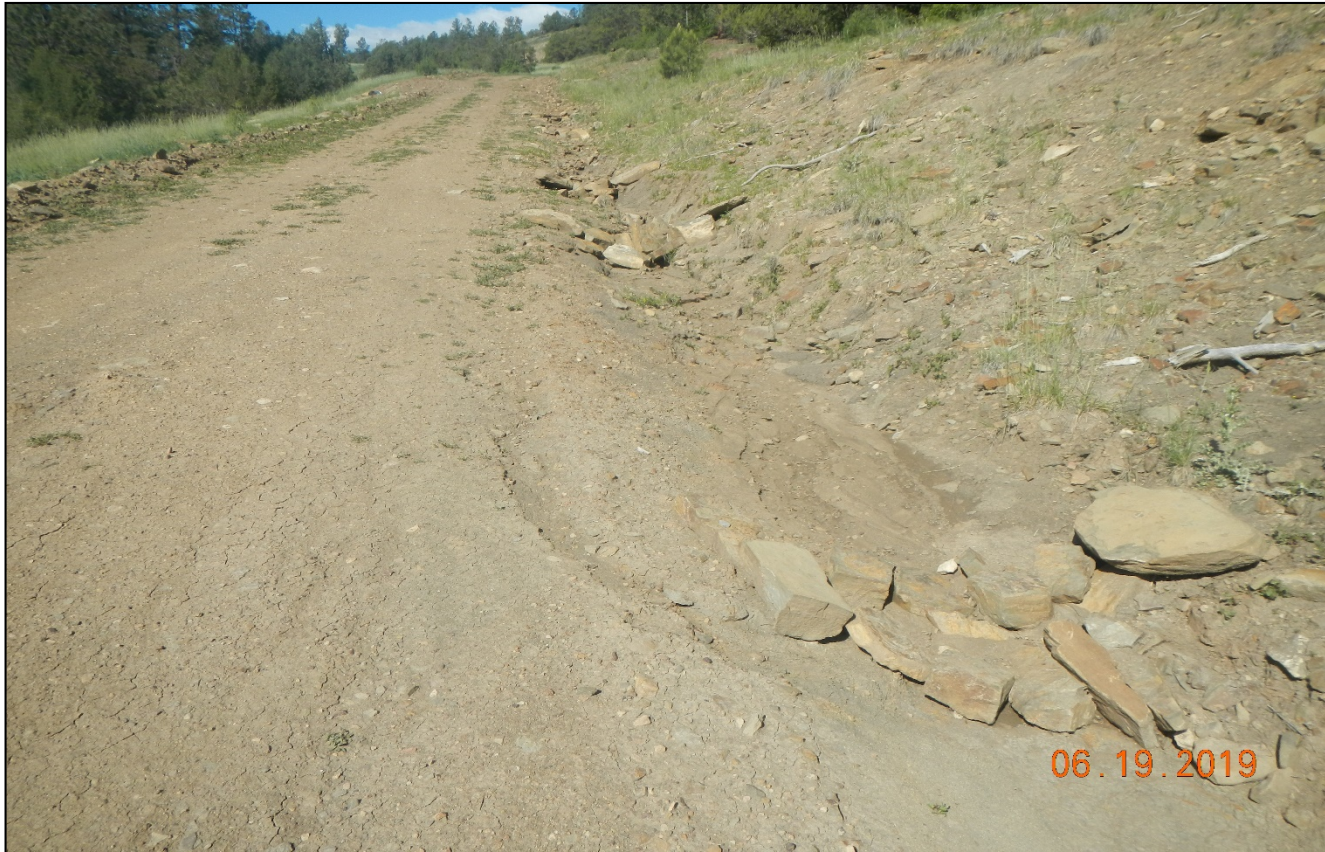
Photo 2. Rock check damns were installed along the side of the access road to the location. Sediment has filled in the check damns or stormwater is flowing around.
