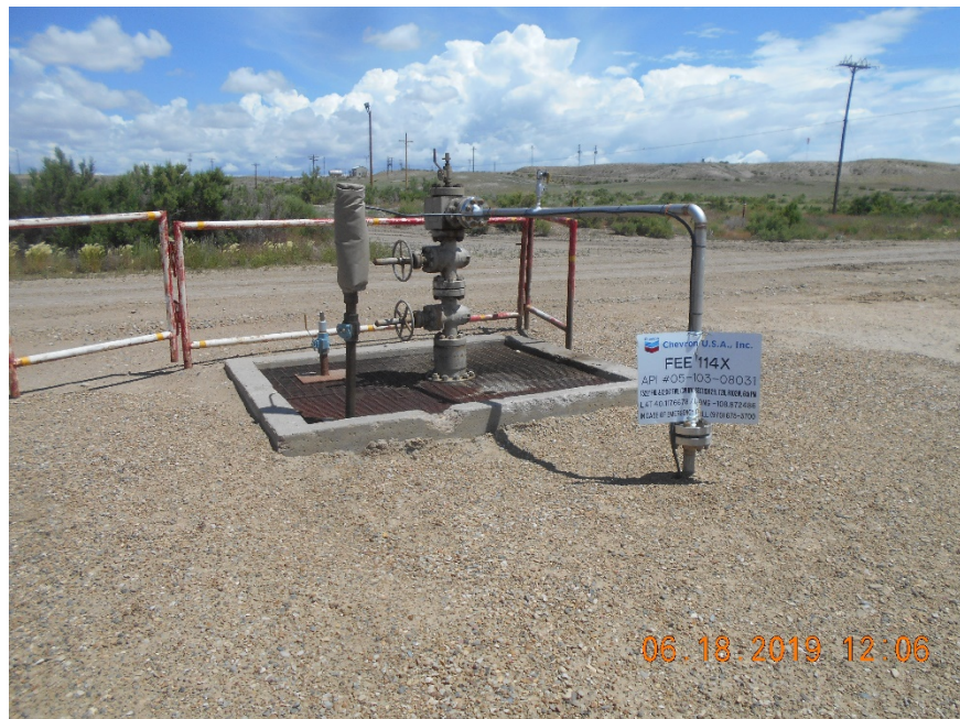
Injection wellhead.
