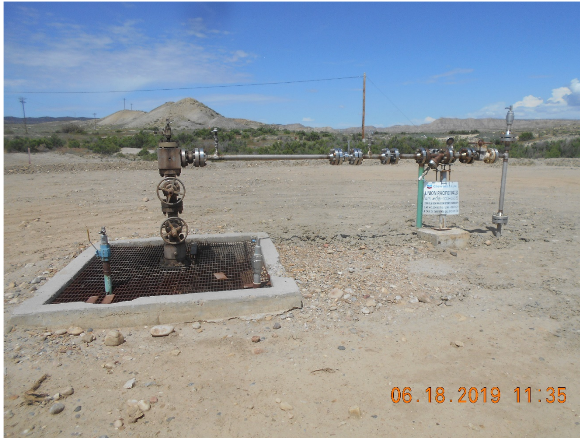
Injection wellhead
