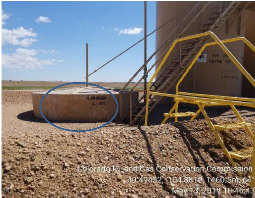
Photo 1: PREVIOUS photo of missing placard on produced water tank
