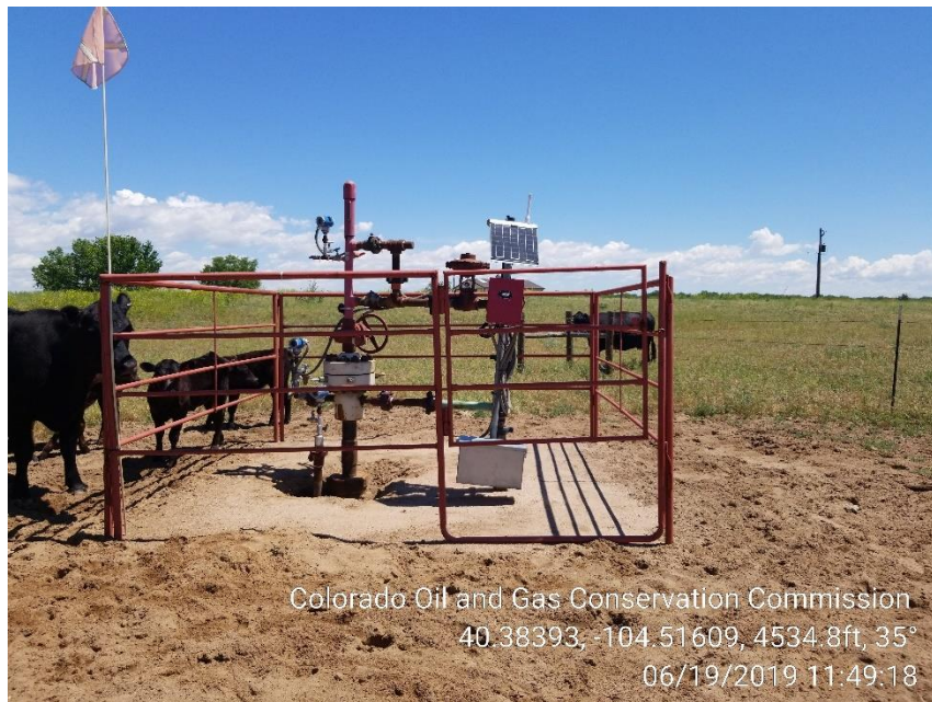
Photo 1 – Chewy B 23-24 Wellhead Sign missing
