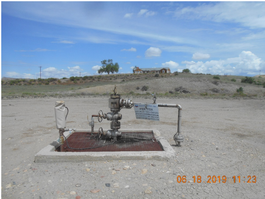
Injection wellhead.
