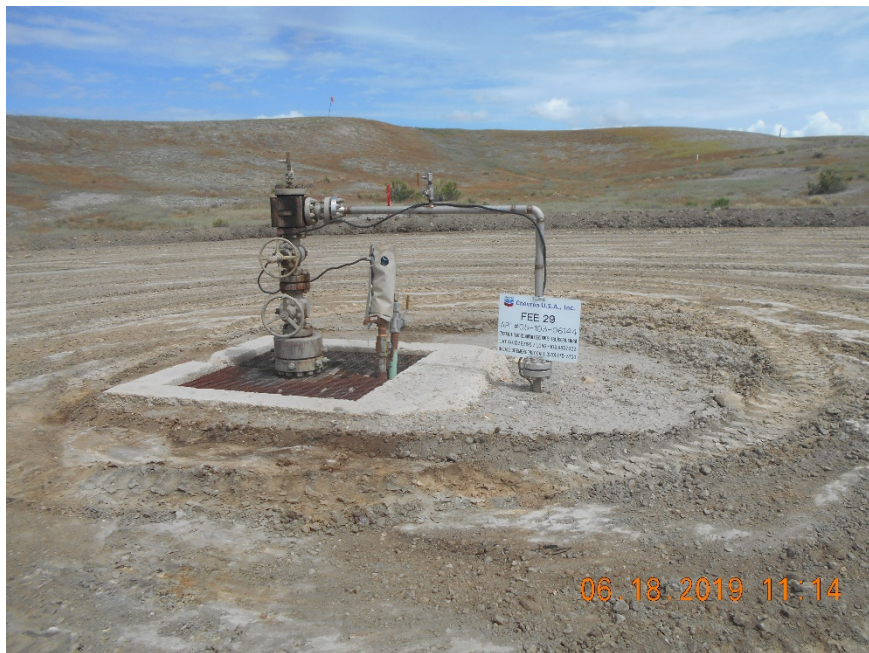
Injection wellhead.
