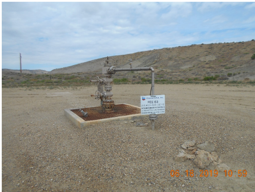
Injection wellhead.
