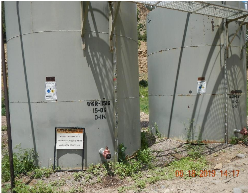
Albert Martinez #1 tank battery. Shared secondary containment berm with Nielson #4.
