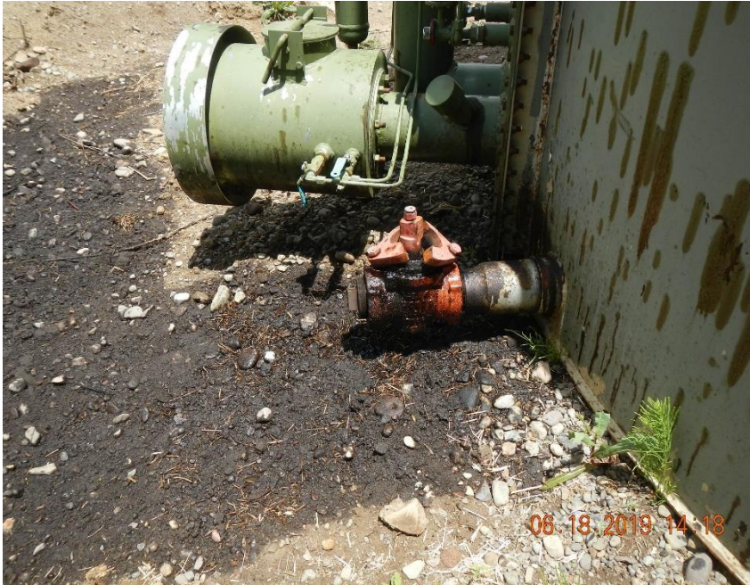
Load out valve on backside of AST is stained and wet.
