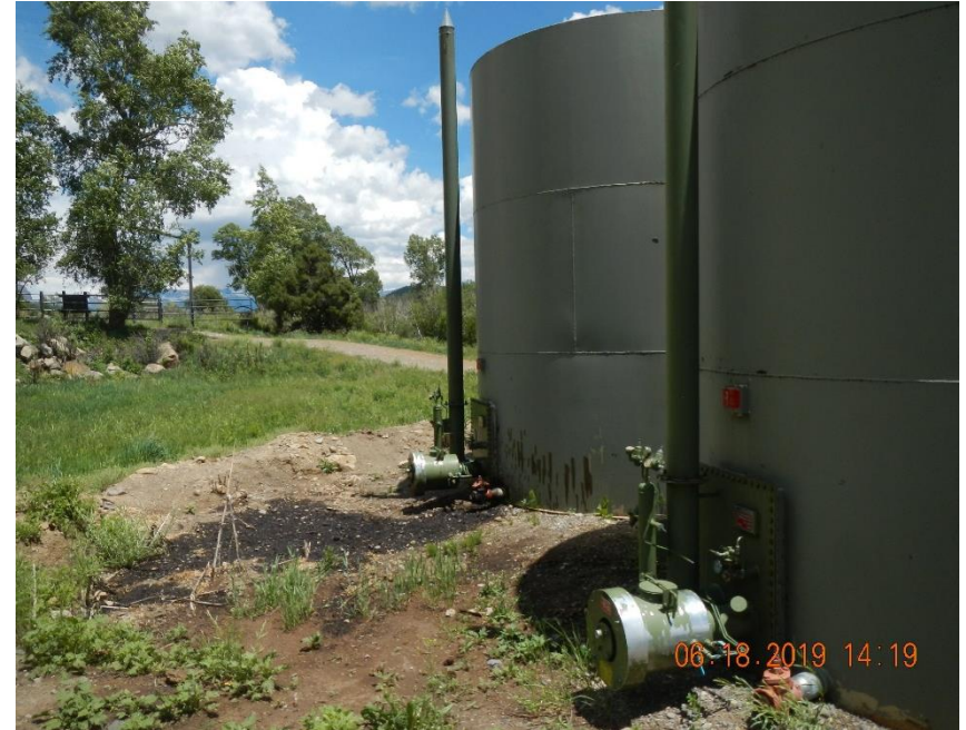
View of crude oil release within secondary containment berm.
