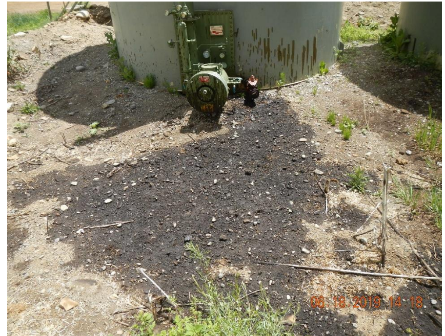
Crude oil release from valve on backside of AST.
