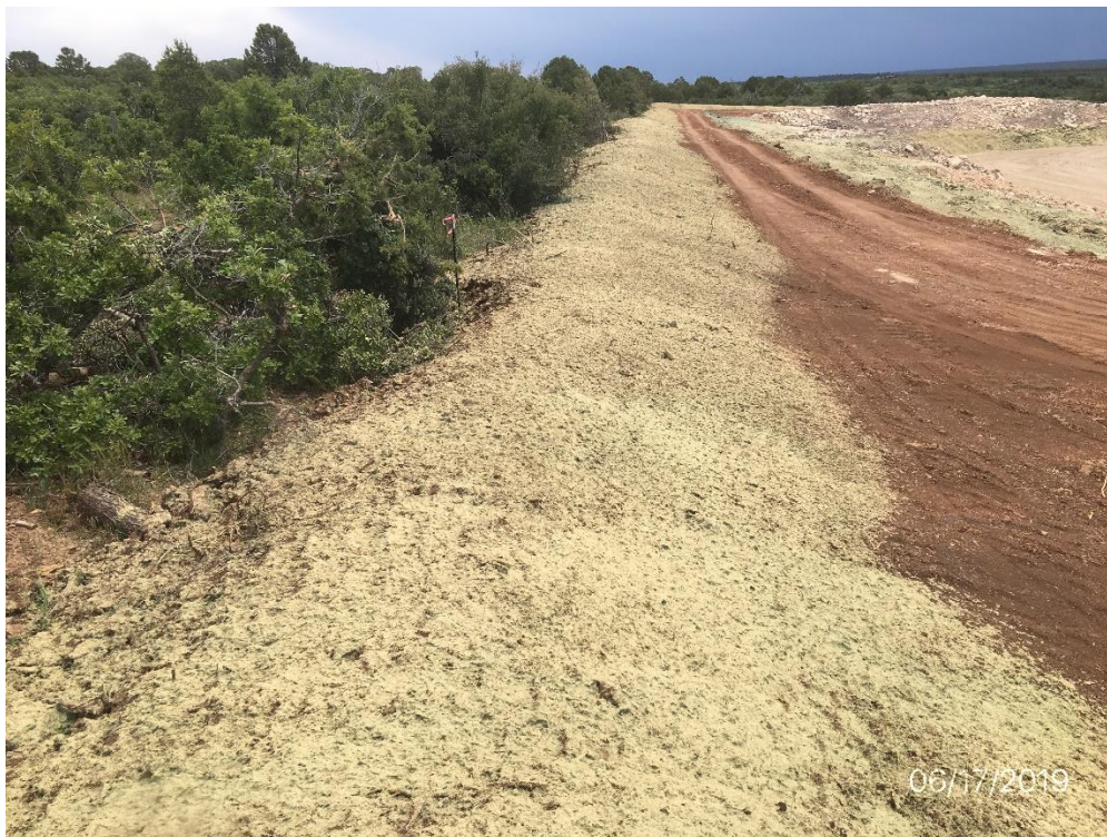
Photo 5: View of the northern project area from the northwestern corner facing eastward. Perimeter controls and erosion controls installed to stabilize bare soils.
