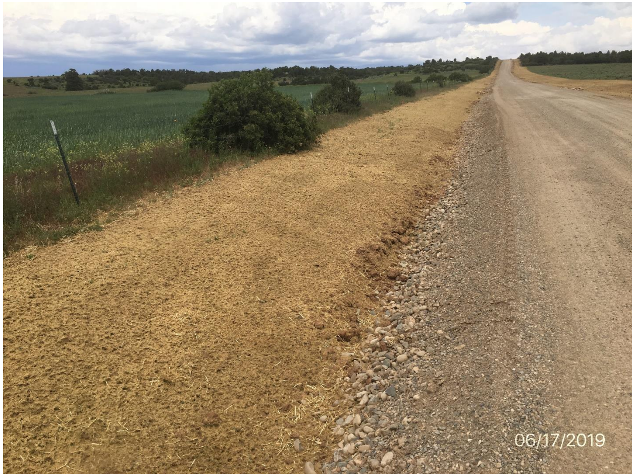
Photo 1: View of storm water perimeter controls along the western edge of the access road.
