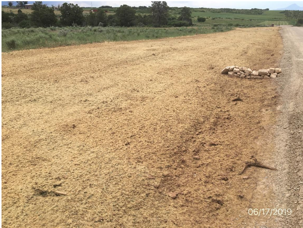
Photo 4: Perimeter controls installed along access road to prevent topsoil loss.
