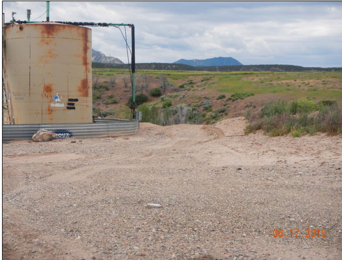
Photo # 5 Berm at SW corner of location need maintenance.
