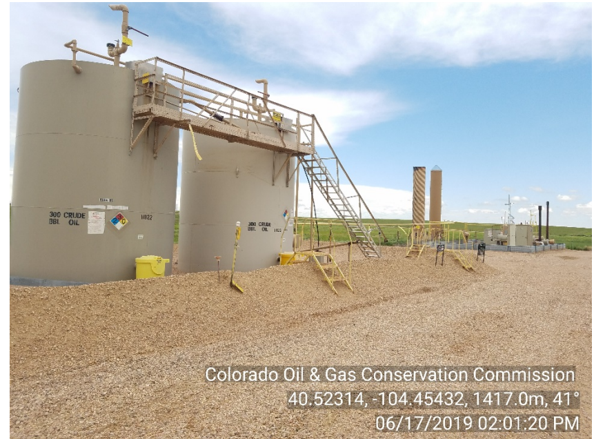
Photo #4 Turman 32-42 Battery Inadequate low berms - Appears Mitigated
