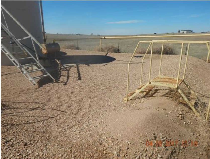
Photo #3 Turman 32-42 Battery Inadequate low berms from prior insp.
