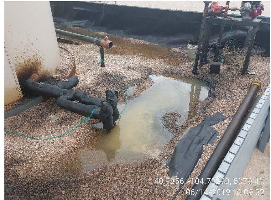
Photo 14 – Stormwater mixed with oil inside AST secondary containment.
