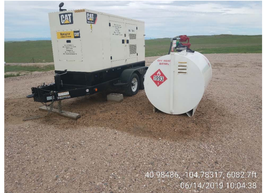
Photo 4 – Diesel AST either leaks or was overfilled. Stain on ground has diesel odor.
