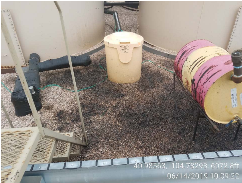
Photo 13 – Residual oil impacts in AST secondary containment.
