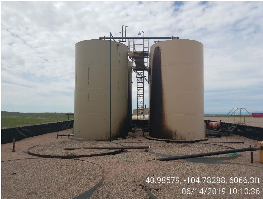
Photo 15 – Oil stains on ASTs from former oil release.
