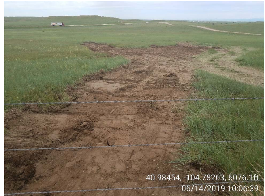
Photo 8 – Spill traveled offsite onto rangeland. Looking south from fence on south edge of pad.
