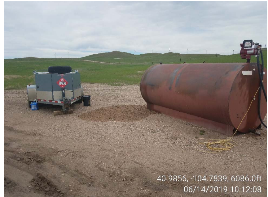
Photo 16 – Diesel fuel leaked from AST stored on northwest corner of location.
