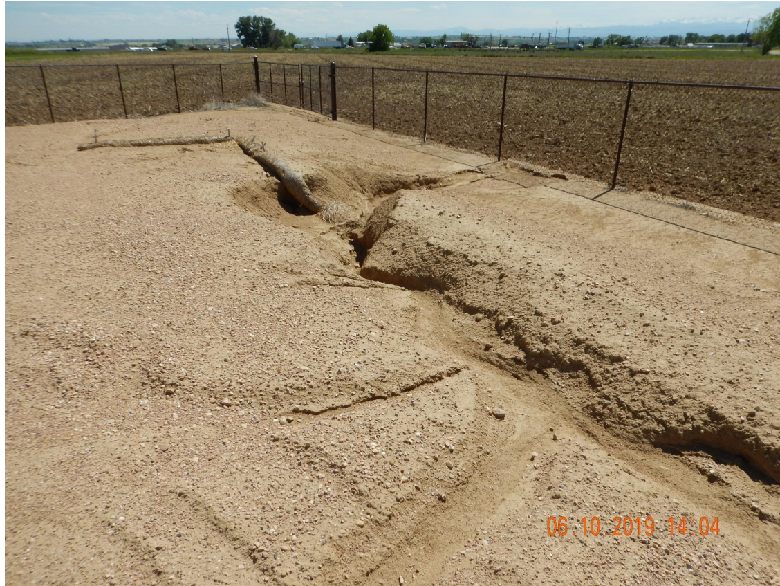
Photo 1. Photo taken from the southwestern location, facing South. Operator has failed to implement long-term stormwater BMPs to prevent sediment laden stormwater from leaving location. Photo illustrates gully erosion with sediment discharge off location.
