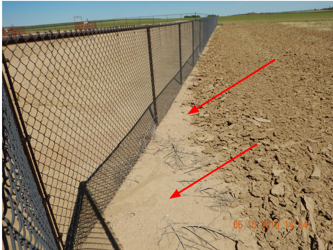
Photo 4. Photo taken from the southern location, facing East. Photo illustrates sediment discharge off location.
