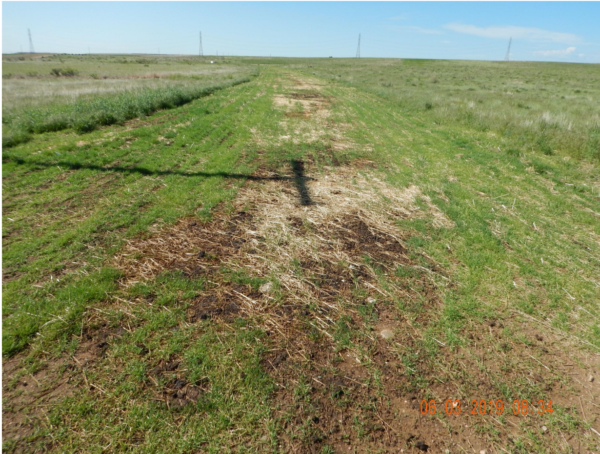
Photo 1. Photo taken from the entrance of the location, facing South. Operator has performed the previous corrective action to perform final reclamation activities at the well location and access road. At the time of this inspection, germination was apparent throughout the access road.
