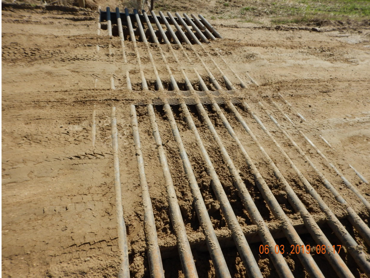
Photo 3. Photo taken from the entrance of location, facing East. Appears maintenance is required as sediment has accumulated in the tracking device BMP and is no longer properly functioning.
