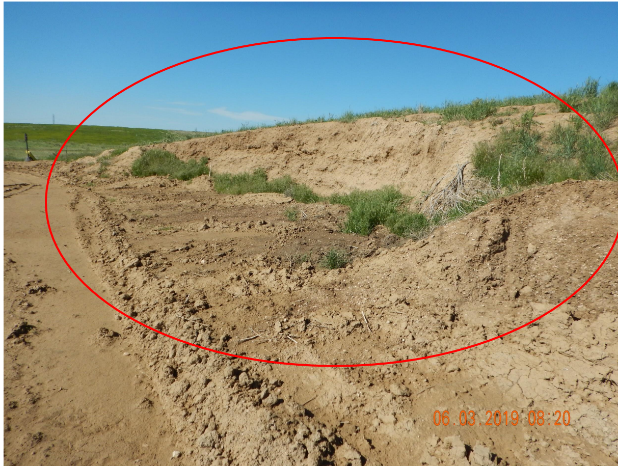
Photo 4. Photo taken from the southern topsoil stockpile, facing South. Appears the Operator has used topsoil but has not yet performed interim reclamation. Topsoil shall only be used to facilitate subsequent reclamation.
