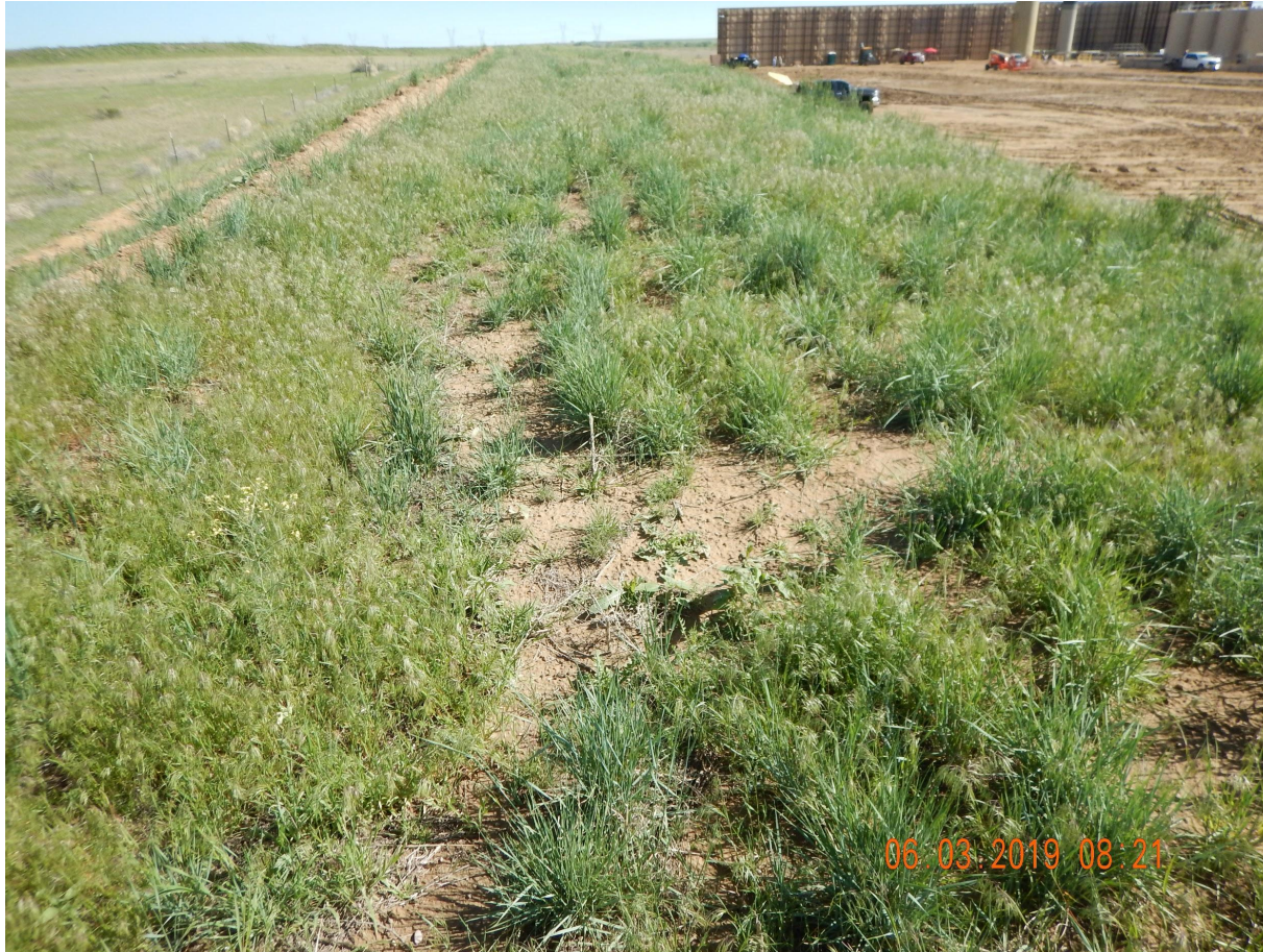
Photo 6. Photo taken from the southern topsoil stockpile, facing North. Operator has failed prevent weed establishment on the topsoil stockpile.
