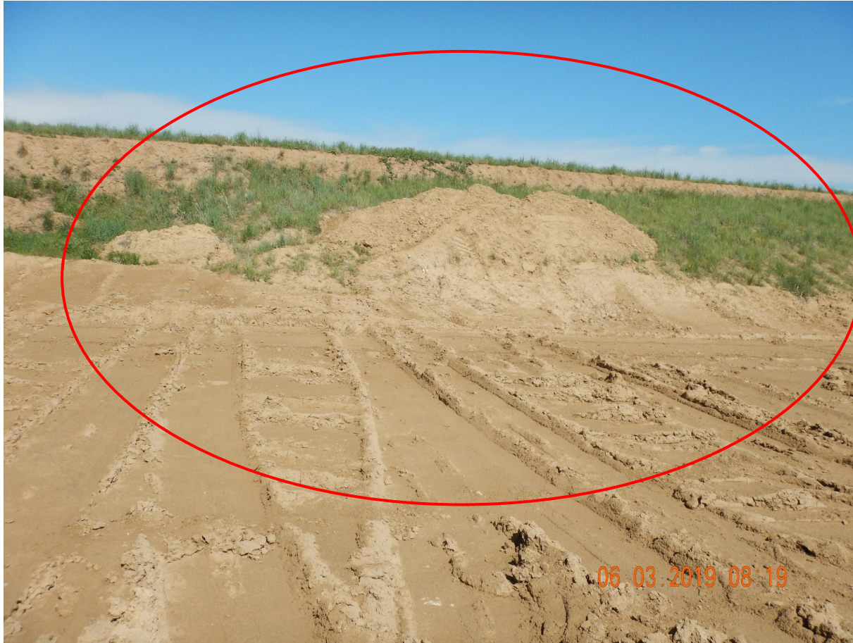
Photo 5. Photo taken from the southern topsoil stockpile, facing West. Appears the Operator has scrapped off material from the well pad and placed it on the topsoil stockpile. Operator shall protect topsoil from degradation due to contamination.
