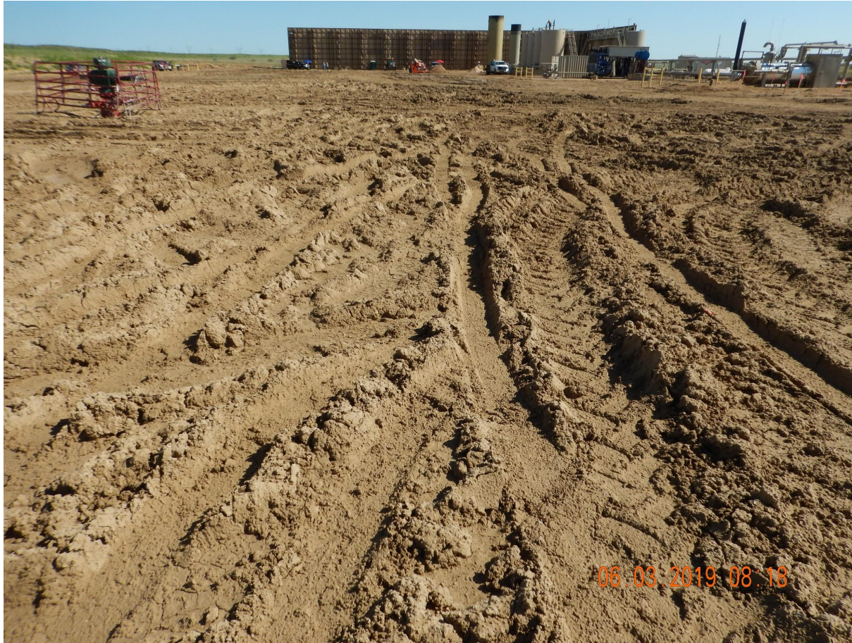
Photo 1. Photo taken from the approximate wellhead, facing North. This location has not been properly constructed and maintained so as to reasonably minimize erosion and removal of surface material. Ruts were over one foot in depth and vehicles are tracking sediment offsite.
