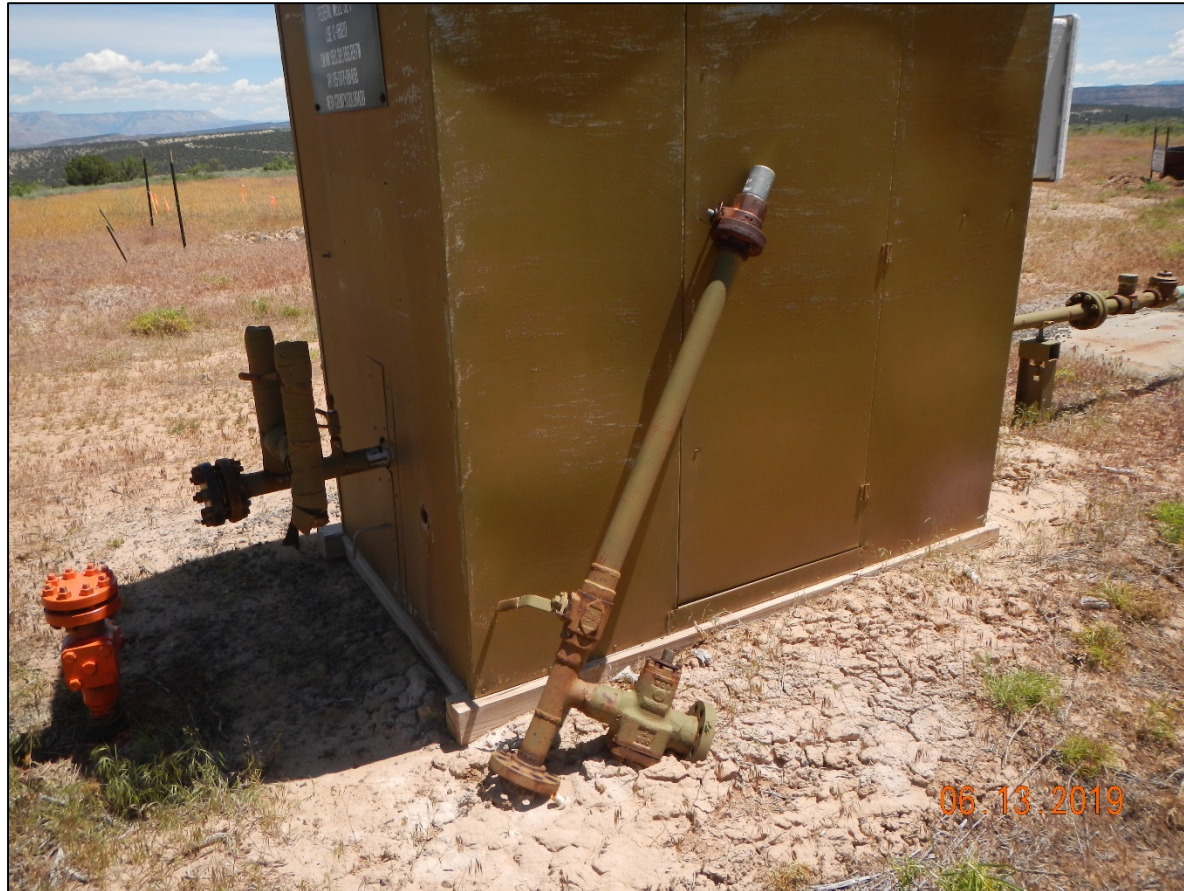
Photo # 6 unused riser left stored on location. Orange Riser not LOTO
