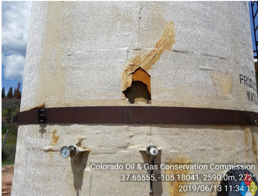
PHOTO 7: THERE IS A HOLE AND SEVERAL CRACKS IN OUTER LAYER OF THE DOUBLE WALL PRODUCED WATER TANK. COMPLY WITH 605 SERIES RULES FOR MECHANICAL CONDITIONS. CA DATE 7/13/19
