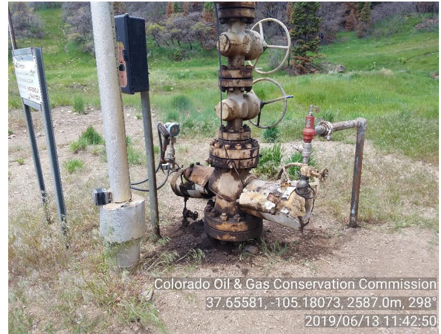
PHOTO 2: IMPACTED SOIL AROUND WELLHEAD. Remove and dispose impacted material in approved manner, service and maintain equipment and self inspect to prevent recurrence of conditions per 1002.f(2) and 907. CA DATE 7/13/19
