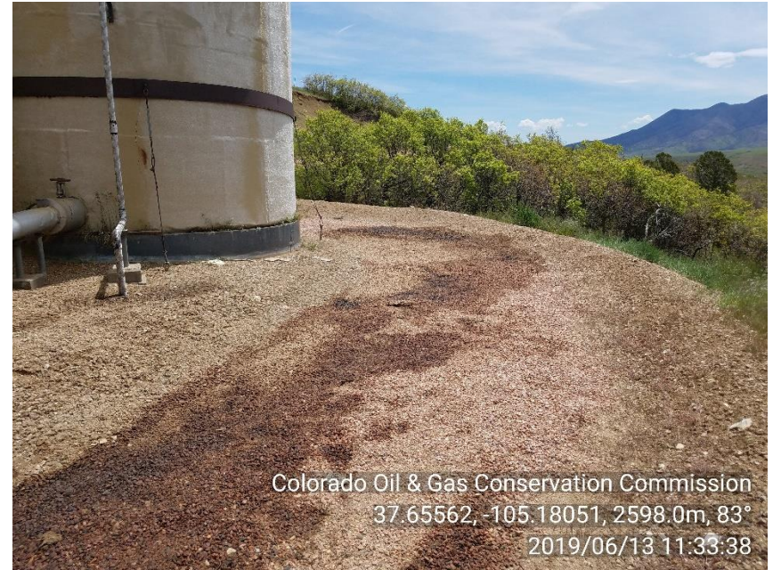
PHOTO 4: IMPACTED SOIL IN CONTAINMENT SOUTHWEST OF PRODUCED WATER TANK. Control and contain spills/releases and clean up per Rule 906.a.CA DATE 7/13/19
