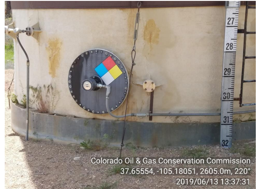
PHOTO 8: HAZARD LEVEL NUMBERS ARE FADED AND NOT LEGABLE ON LARGER PRODUCED WATER TANK (SOUTHEAST TANK). ALSO CAPACITY OF TANK IS NOT POSTED. COMPLY WITH 210 SERIES RULES. 7/13/19
