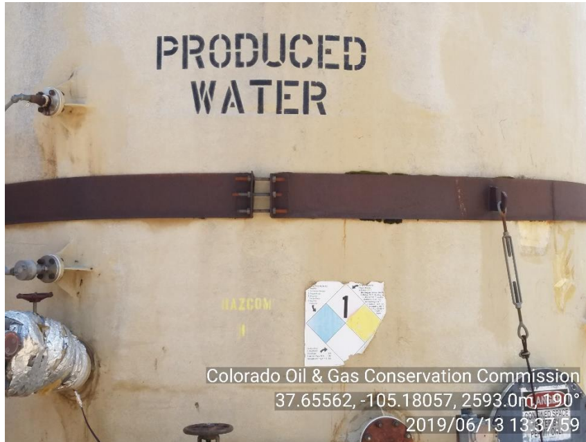
PHOTO 9: CAZARD LEVEL NUMBERS ARE FAIDED AND NOT LEGABLE ON LARGER PRODUCED WATER TANK (SOUTHEAST TANK). ALSO CAPACITY OF TANK IS NOT POSTED. COMPLY WITH 210 SERIES RULES. 7/13/19
