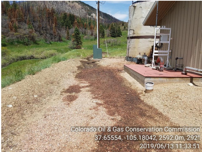
PHOTO 5: IMPACTED SOIL IN CONTAINMENT SOUTH OF OIL TANK. Control and contain spills/releases and clean up per Rule 906.a.CA DATE 7/13/19
