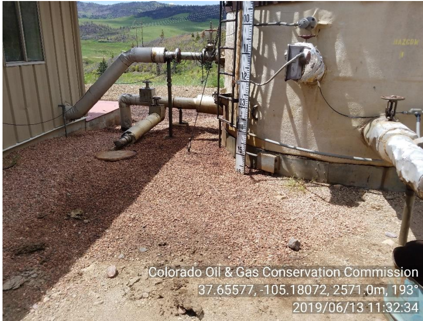
PHOTO 3: IMPACTED SOIL AROUND OIL TANK. Control and contain spills/releases and clean up per Rule 906.a.CA DATE 7/13/19
