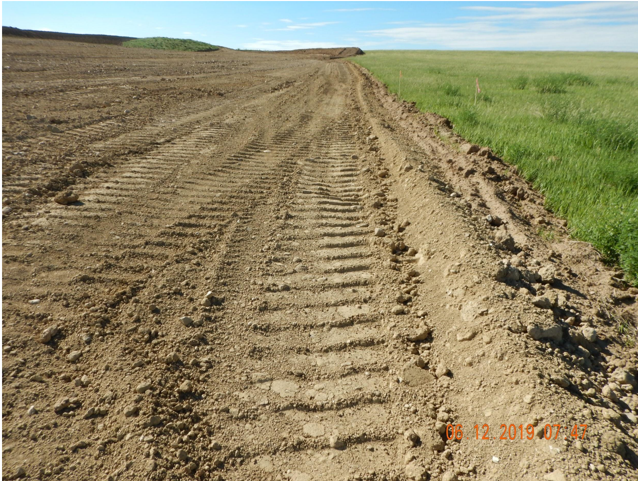
Photo 3. Photo taken from the northwestern perimeter of location, facing South. Photo illustrates the Operator is performing construction activities (i.e., interim reclamation) and has failed to install perimeter BMPs.
