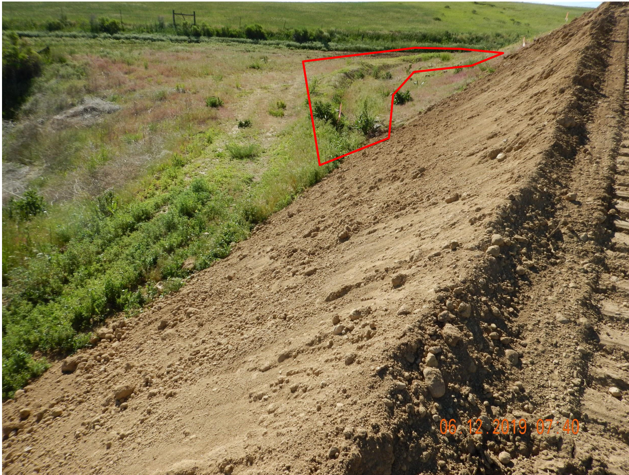
Photo 6. Photo taken from the northeastern perimeter of location, facing East. Photo illustrates soil material has covered up the previous ditch and berm (highlighted in red) and has failed to install perimeter BMPs.
