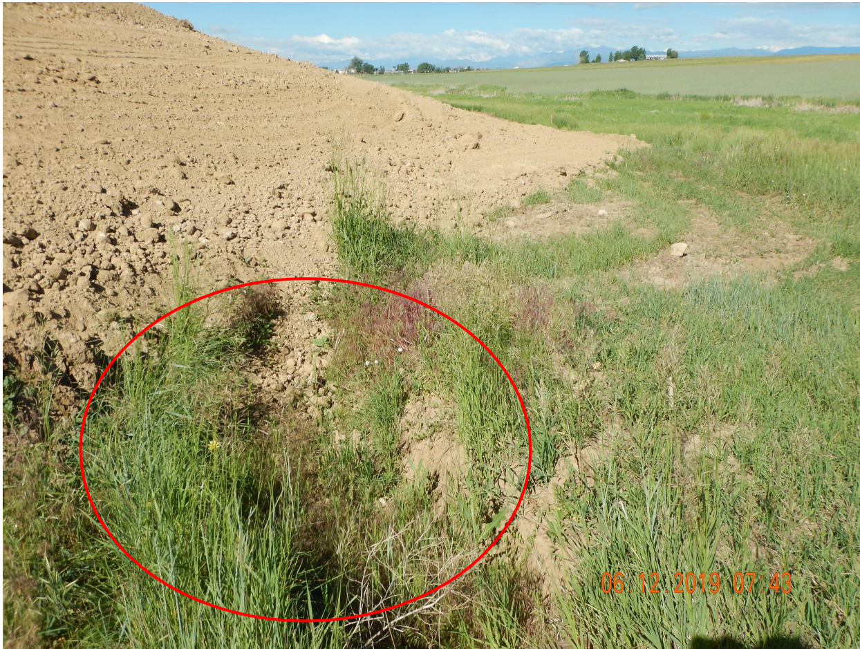
Photo 5. Photo taken from the northeastern perimeter of location, facing West. Photo illustrates the ditch and berm BMP that was previously installed during initial construction activities; however, the Operator has failed to install perimeter BMPs for other portions of the disturbance area.
