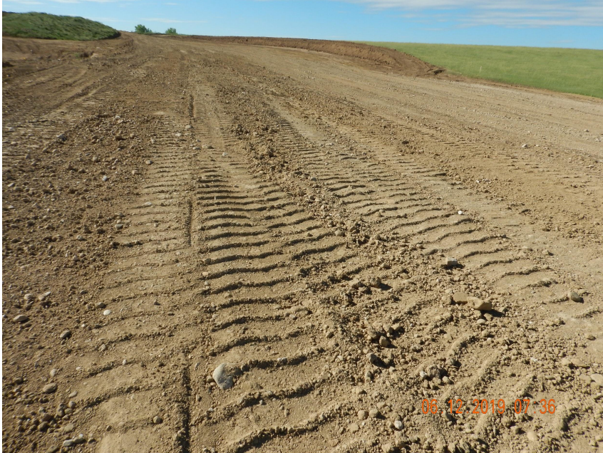
Photo 1. Photo taken from the western interim reclamation area, facing South. Operator is in-process of performing interim reclamation activities. The previous corrective action for erosion on the fill slopes has been mitigated by reducing the steepness by extending the location outward.
