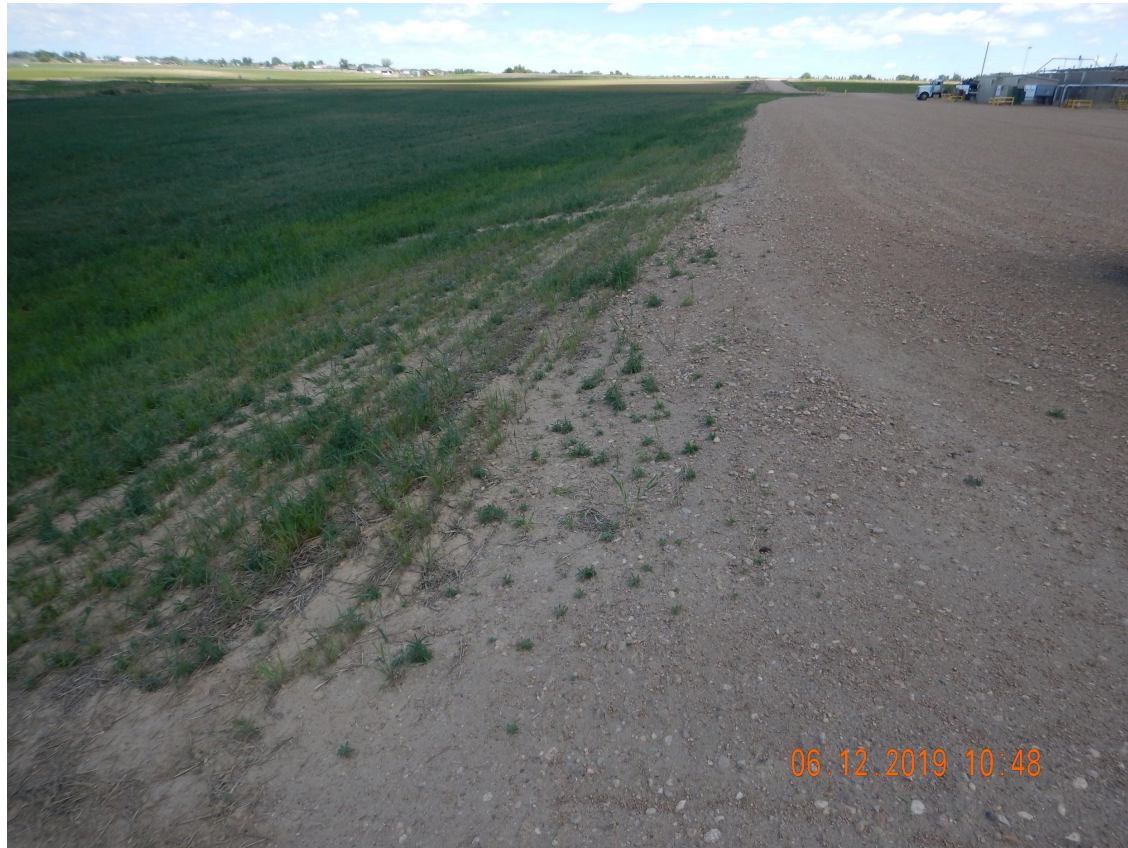
Photo 5. Photo taken from the southwestern location, facing North. Operator has only made repairs to the erosion but has not implemented additional BMPs to prevent sediment laden stormwater from leaving location. Sediment laden stormwater will continue to leave the Location because the Operator has not implemented sufficient long-term stormwater BMPs.
