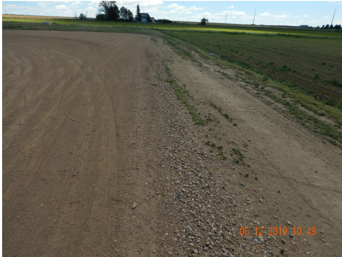
Photo 4. Photo taken from the southern location, facing East. Operator has made repairs to the erosion but the fill slope has not been properly stabilized. Appears the southern fill slope has been seeded but there was no observed mulch or other BMP to stabilize the fill slope until successful germination or establishment of vegetation.
