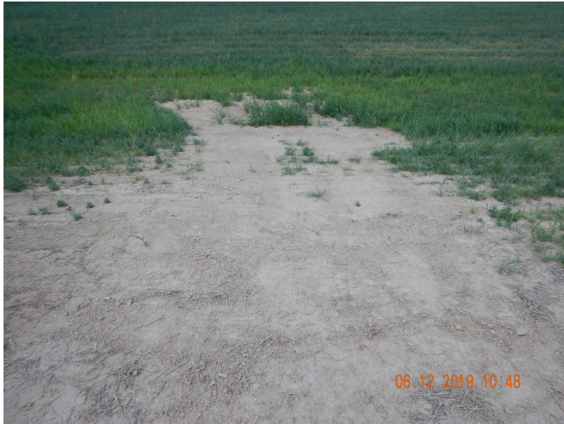
Photo 3. Photo taken from the southwestern location, facing West. Operator has made repairs to the erosion but the fill slope has not been properly stabilized. Straw mulch and germination was observed throughout portions of the western fill slope- see Photo 5- but not where erosion was repaired.
