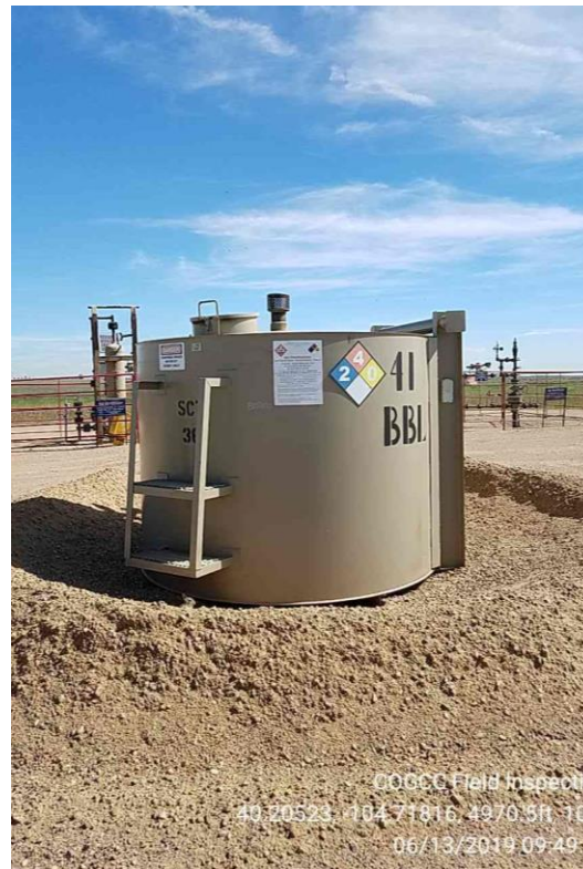
Photo 2 Bradenhead monitoring tank
