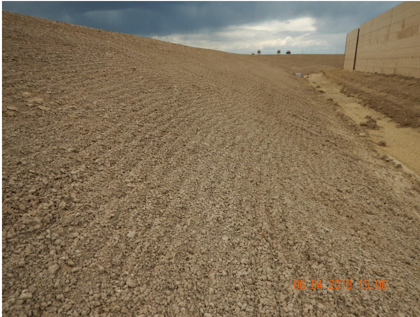
Photo 3. Photo taken from the eastern cut slope from the location, facing South. Operator has temporarily stabilized the cut slope with equipment tracking.
