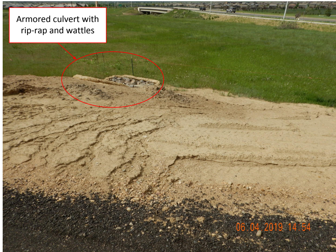
Photo 11. Photo taken from the exit of location, facing North. Fill slopes along the access road have not been properly stabilized and there are no perimeter BMPs in place to mitigate potential sediment laden stormwater from leaving the access road. Photo illustrates rill erosion occurring along the northern fill slope.
