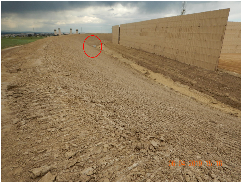
Photo 7. Photo taken from southwestern ridge of location, facing North. Fill slope areas have been temporarily stabilized with equipment tracking. Photo also illustrates what appears to be a retention area with an outlet (red circle).
