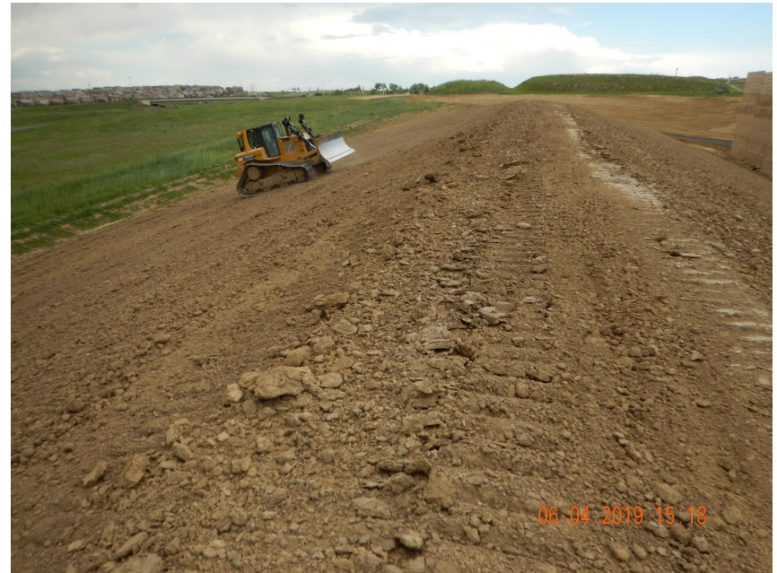
Photo 10. Photo taken from northern ridge of location, facing East. Photo illustrates the Operator temporarily stabilizing the fill slope with equipment tracking.
