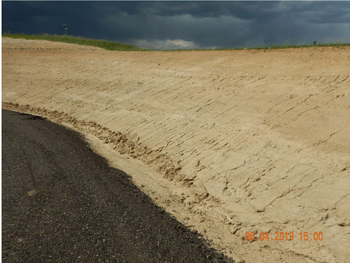
Photo 1. Photo taken from the access entrance of location, facing North. Cut slope has not been properly stabilized on either side of the access road. Photo illustrates rill erosion occurring on the north cut slope.
