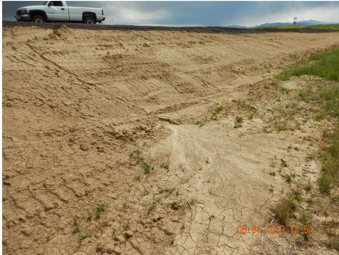
Photo 12. Photo taken from the exit of location, facing South. Fill slopes along the access road have not been properly stabilized and there are no perimeter BMPs in place to mitigate potential sediment laden stormwater from leaving the access road. Photo illustrates sediment leaving the fill slope of the access road with no stormwater BMPs implemented.
