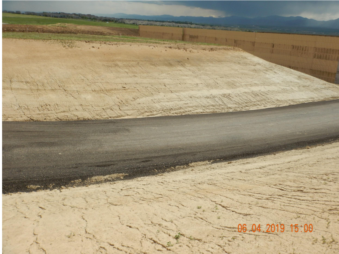
Photo 2. Photo taken from the north cut slope along the access entrance to location, facing South. Cut slope has not been properly stabilized on either side of the access road. Photo illustrates rill erosion occurring on the south cut slope.
