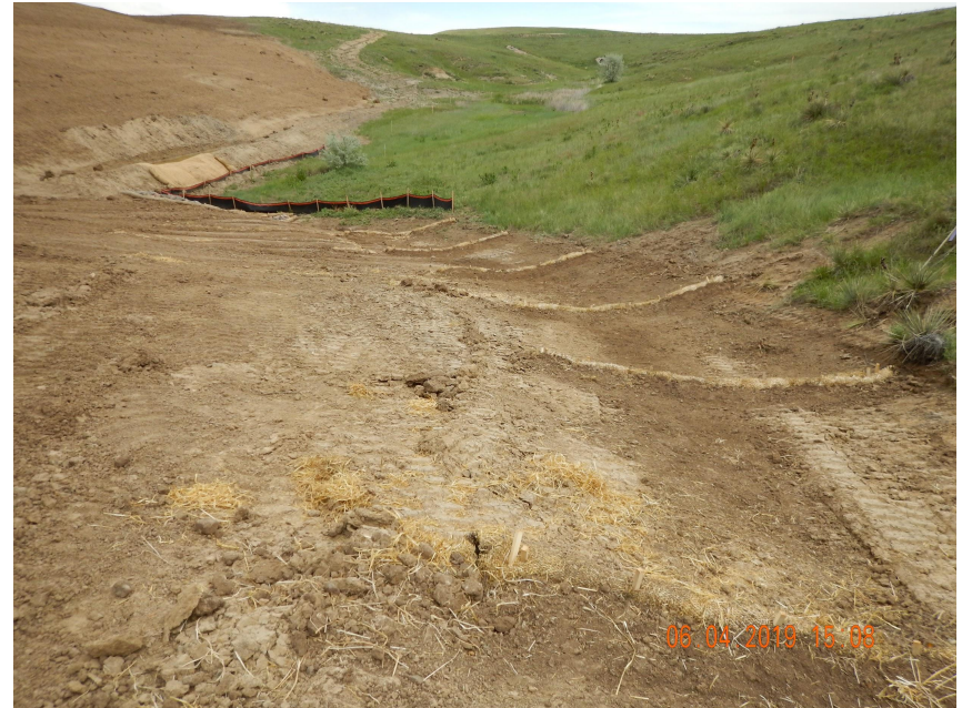
Photo 4. Photo taken from the southwestern perimeter of location, facing Southeast. Operator has installed straw wattles, silt fence and a sediment trap with a temporarily stabilized outlet. All the south-facing fill slopes were temporarily stabilized with equipment tracking.
