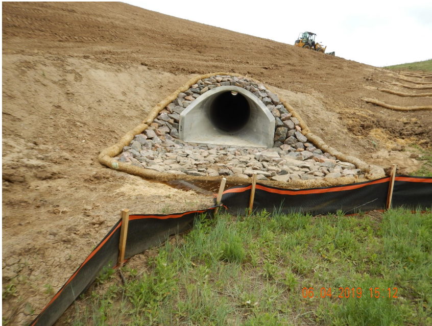
Photo 5. Photo taken from another southwestern portion along the perimeter of location, facing Southeast. Operator has installed a culvert, in conjunction with rip-rap, wattles and silt fence. Operator was repairing silt fence at the time of this inspection.
