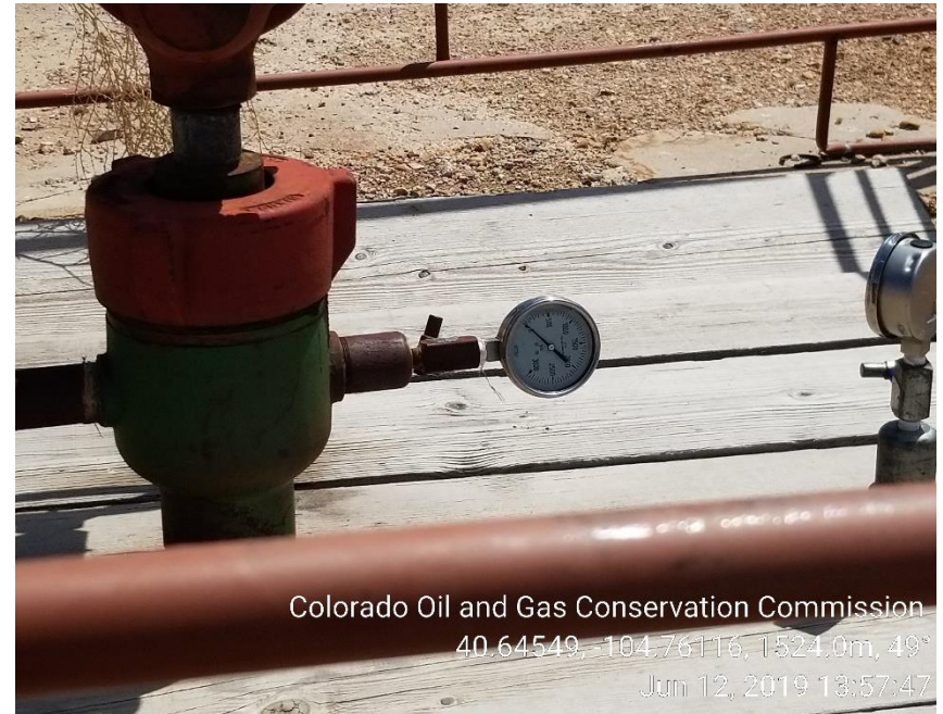
Photo 6: Casing PSI at 0
