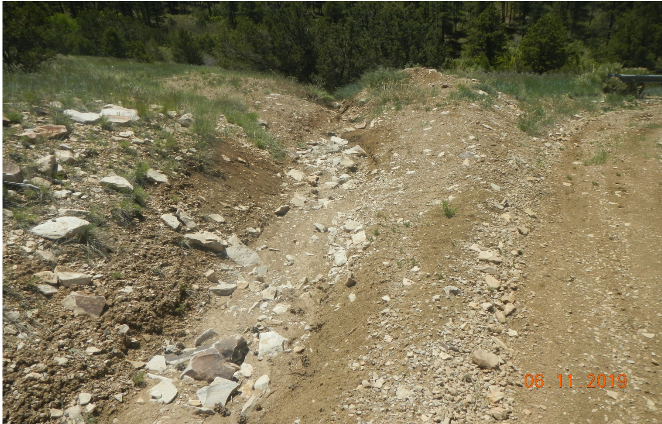
Photo 5. There is no erosion control BMPs at the diversion along the main road. Lat/Long:37.69860,-105.21673
