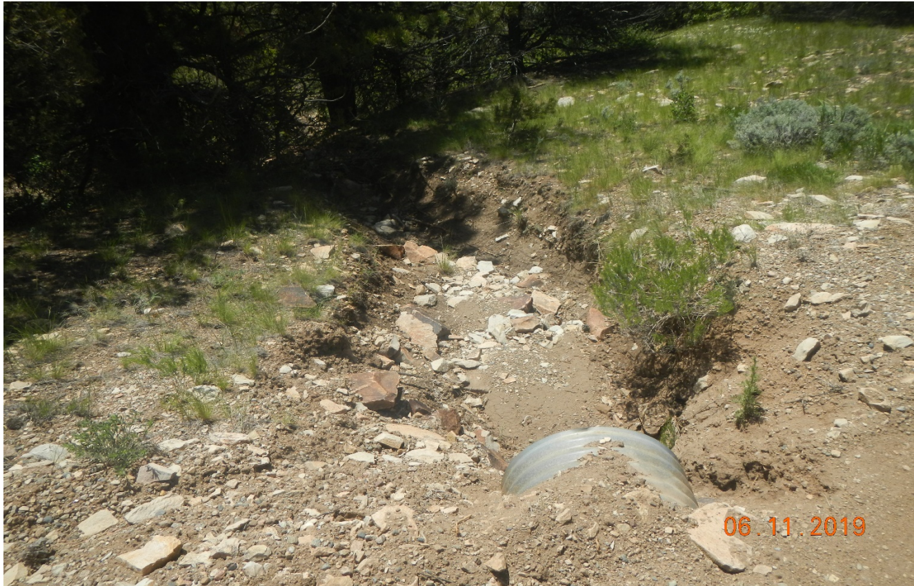
Photo 6. There is erosion occurring at the culvert with no outlet protection. Lat/Long:37.70004,-105.21143
