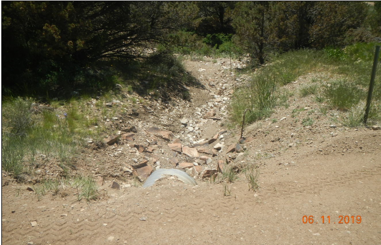
Photo 1. There is erosion occurring at the culvert with no outlet protection. Lat/Long:37.69957,-105.22668
