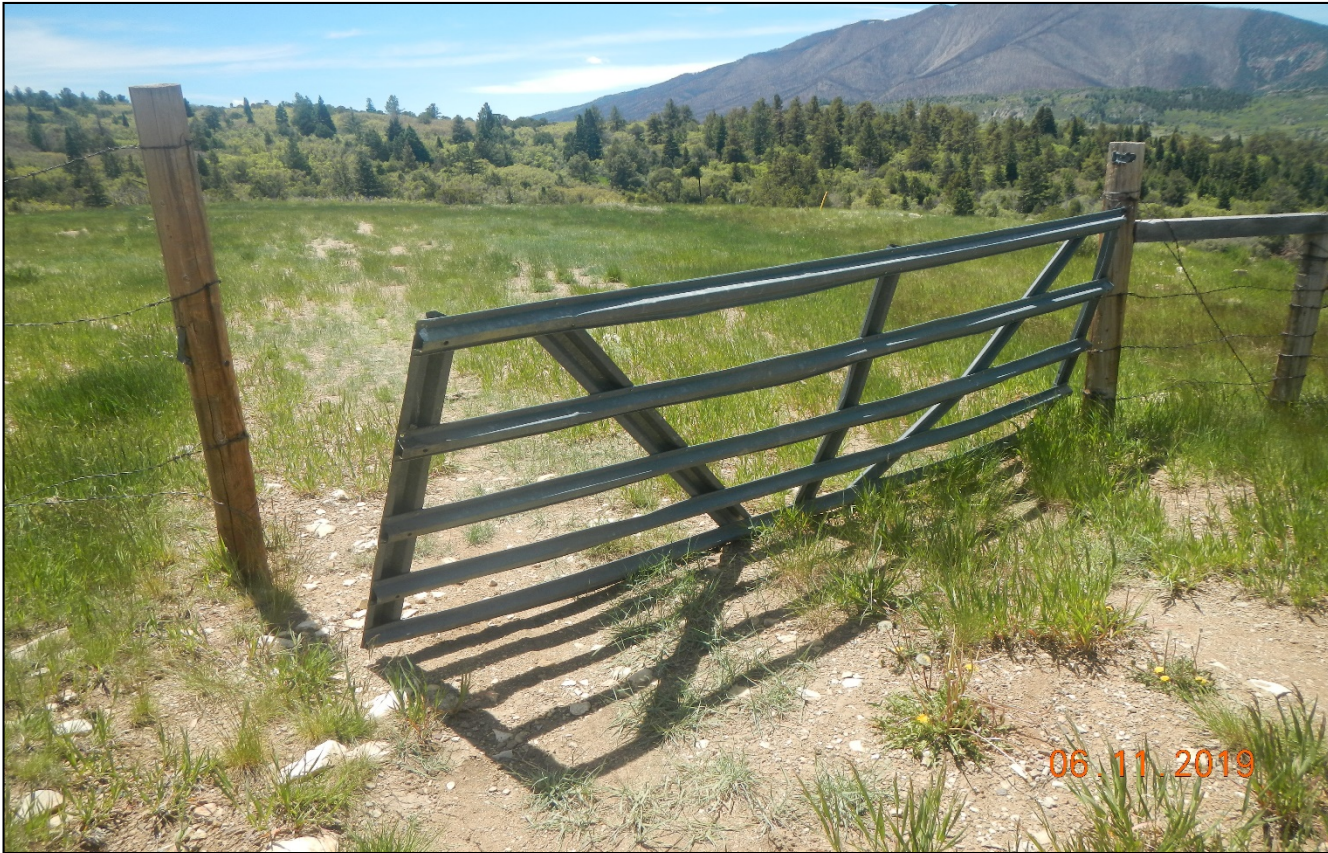
Photo 8. The gate at the location is off the hinges.
