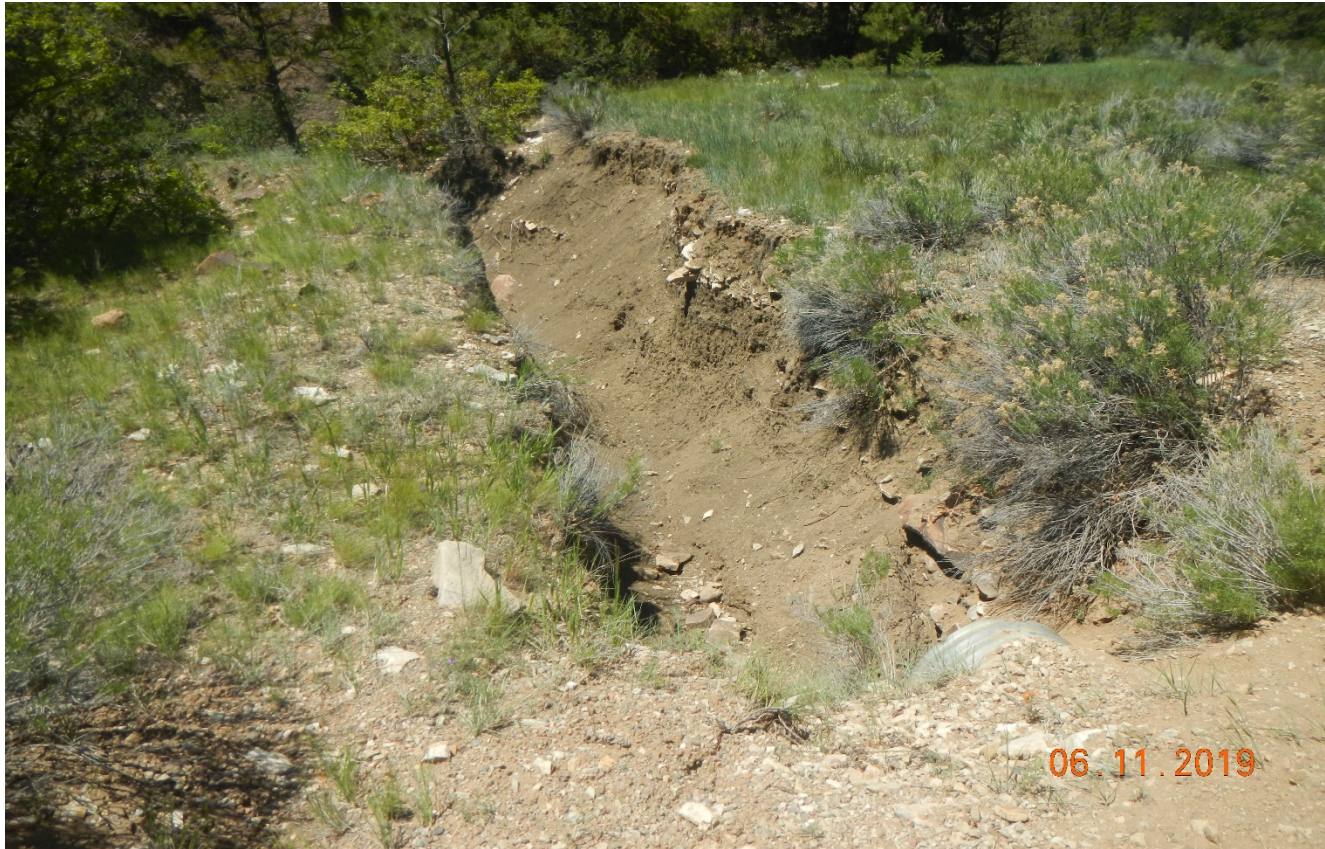
Photo 3. There is severe erosion (6ft. Deep) occurring at the culvert with no outlet protection. Lat/Long:37.69829,-105.21889
