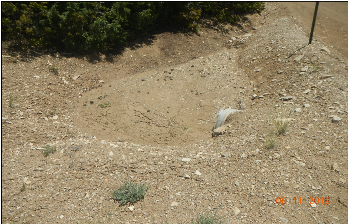
Photo 2. There is sediment accumulating at the culvert inlet.
